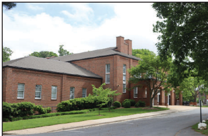
Figure 40: The Mondzac Performing Arts Center was built in 1989. It is located in the northwest section of the Landon School campus. EHT Tracerics.
