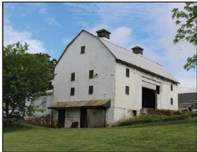
Figure 12: The bank barn that was part of the Lansdale farm. EHT Tracerics.
