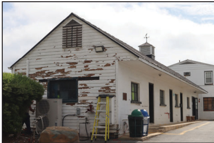
Figure 36: Foster Maintenance Building. EHT Traceries.
