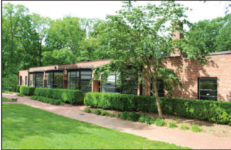
Figure 24: Lower School Building. EHT Traceries.
