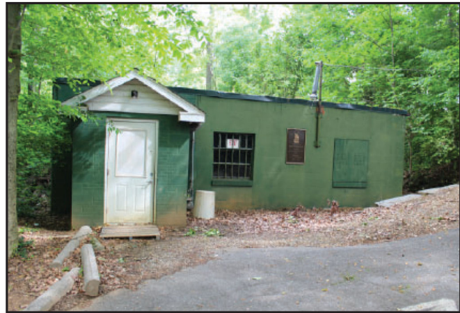
Figure 32: The Frank Parsons Rifle Range. EHT Traceries.
