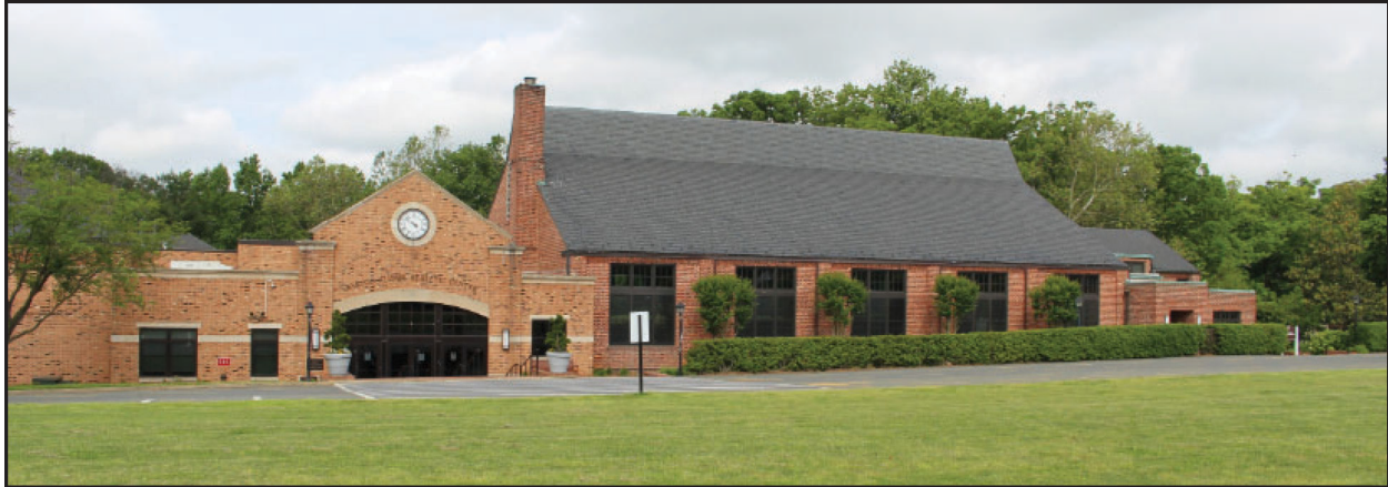
Figure 21: The Barton Alumni Athletic Center. The original 1939 Perkins Gymnasium is visible in the center of the photo with the slate roof. EHT Traceries
