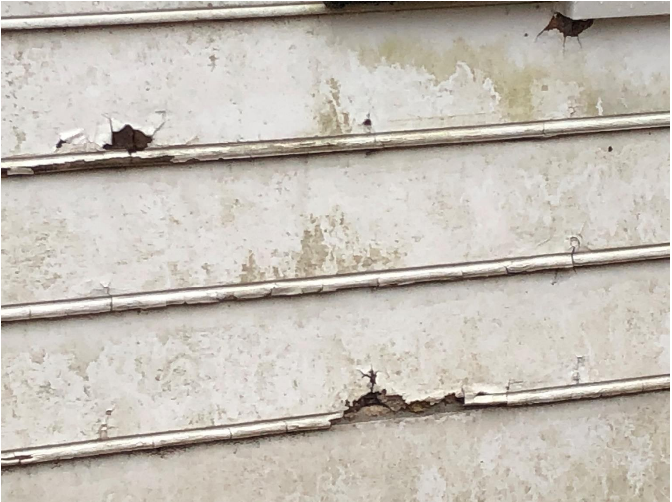
Figure 5: Deteriorated siding on addition (detail)
