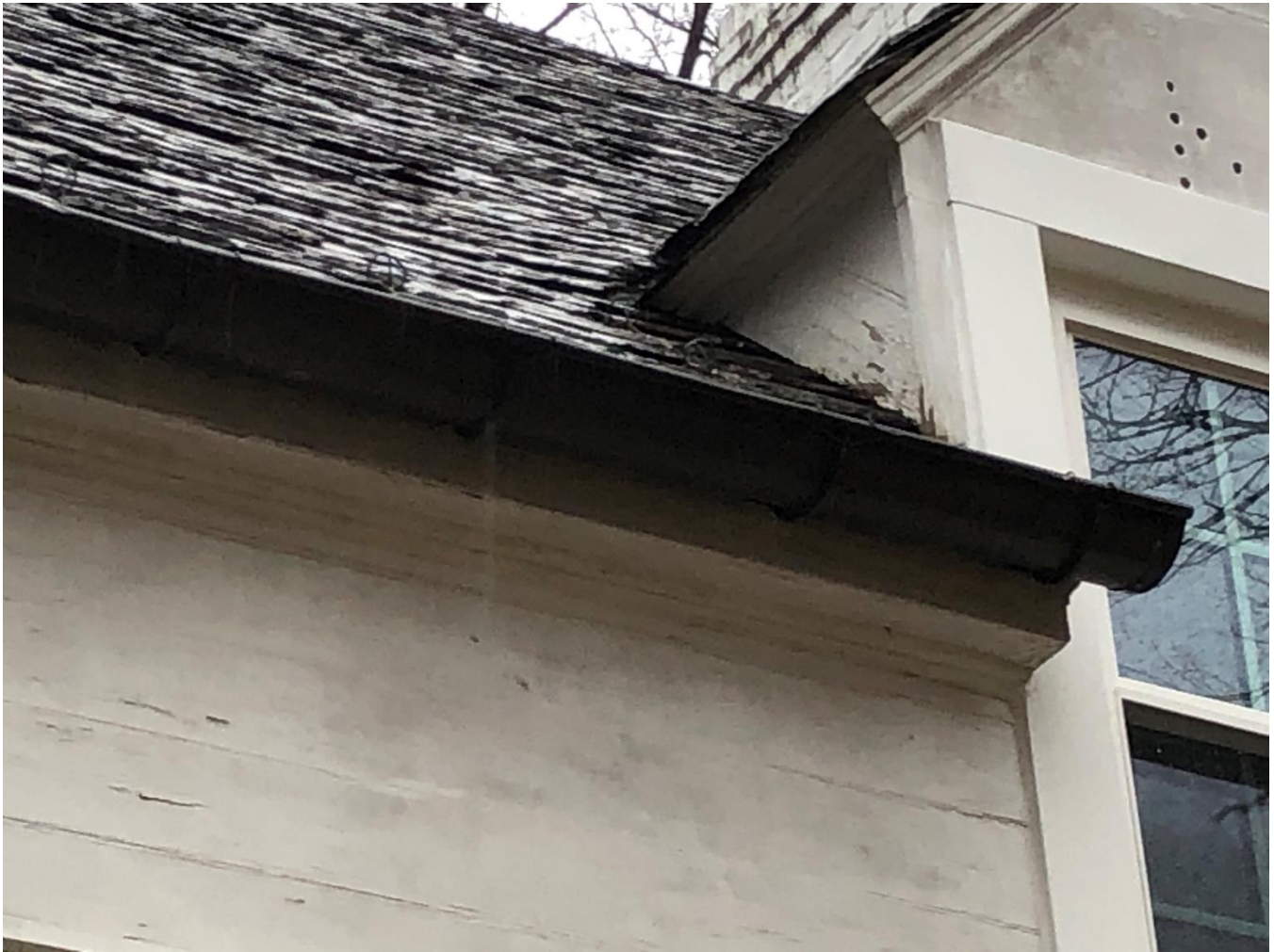
Figure 10: Deteriorated wood siding on dormers
