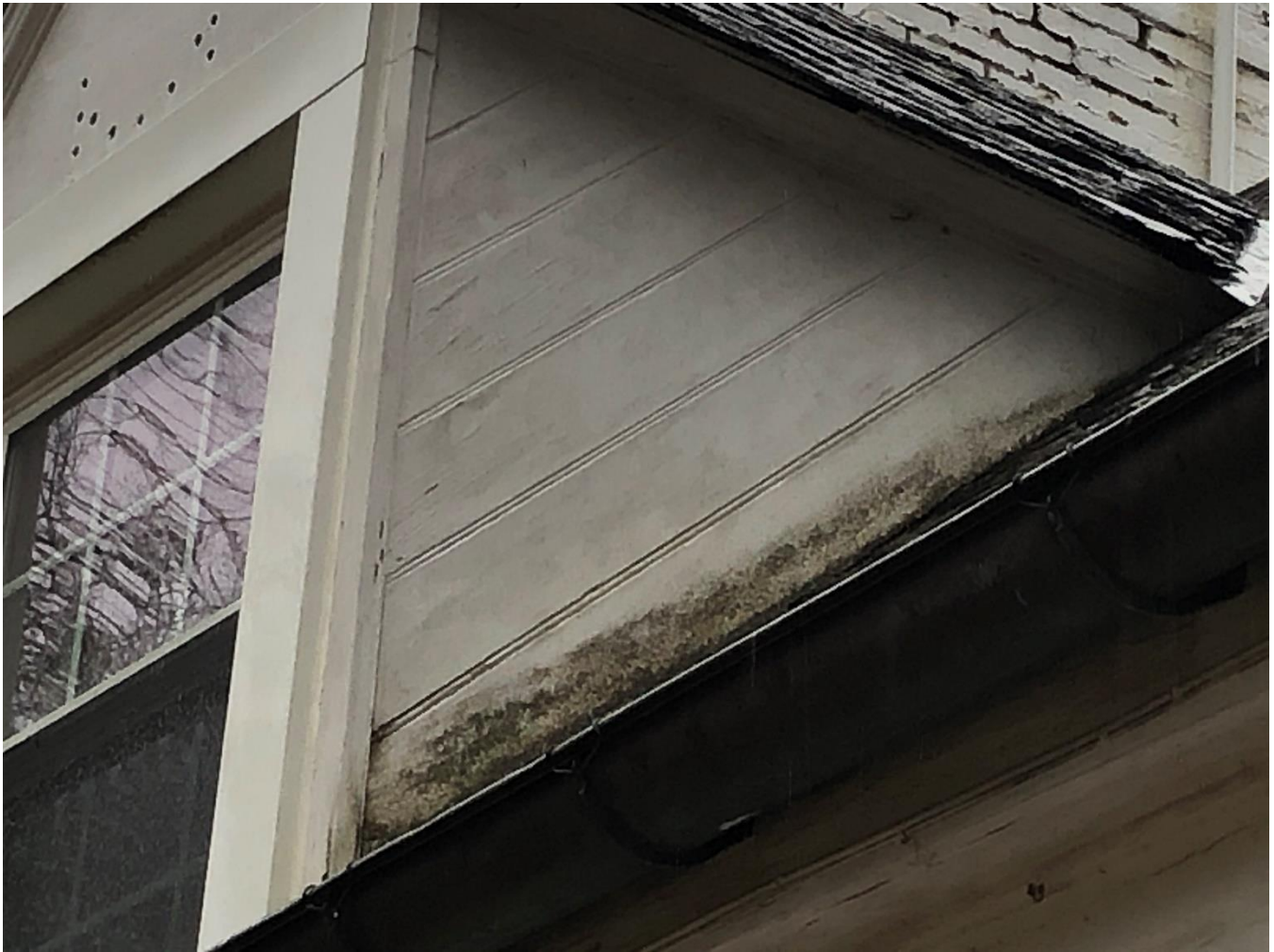
Figure 9: Deteriorated wood siding on dormers (detail)
