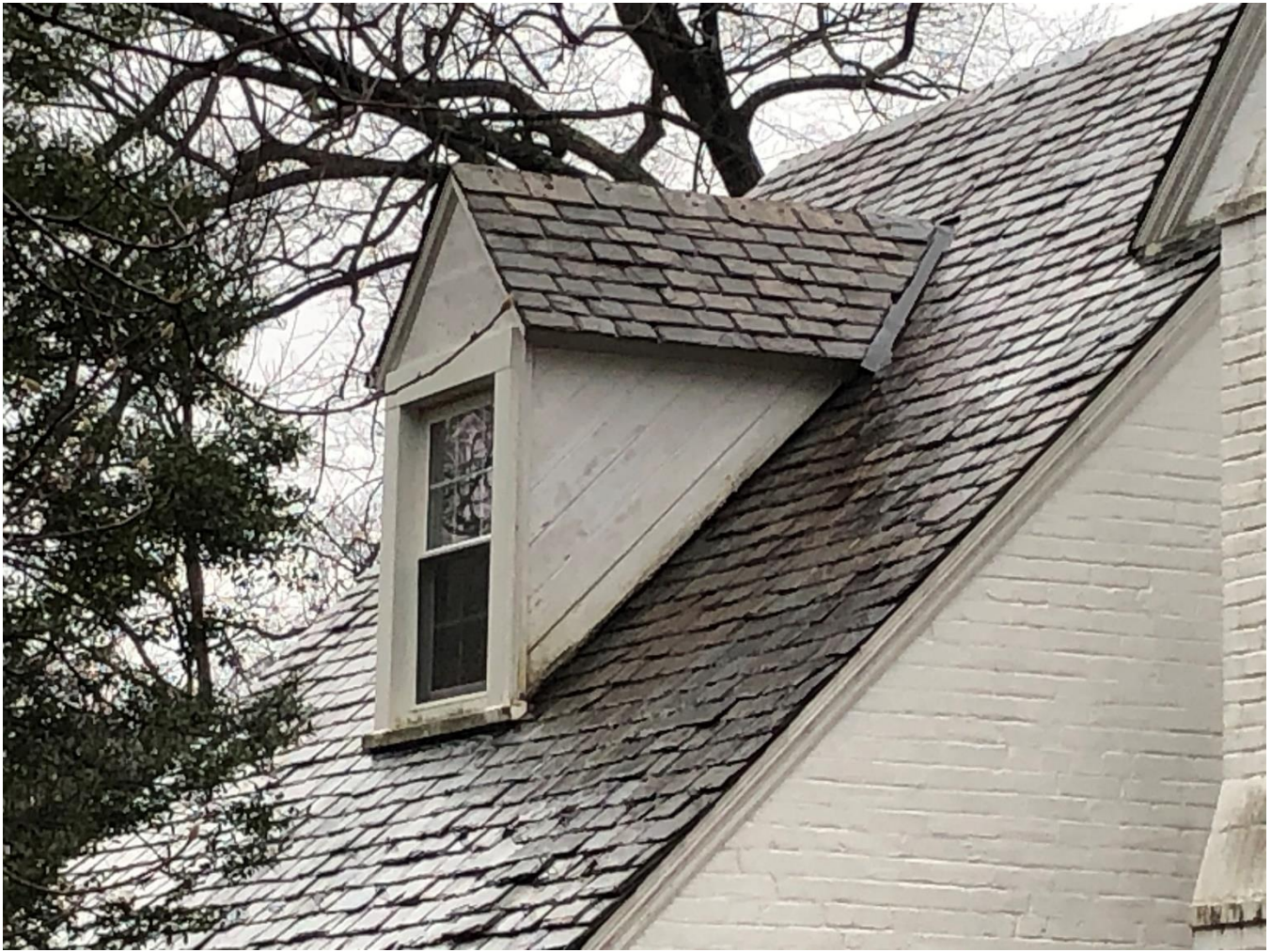
Figure 8: Deteriorated wood siding on dormers
