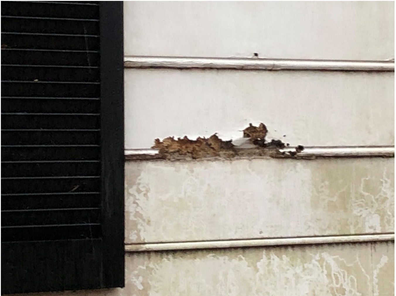
Figure 3: Deteriorated siding on addition (detail)
