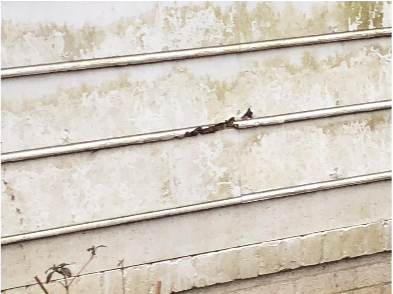
Figure 4: Deteriorated siding on addition (detail)
