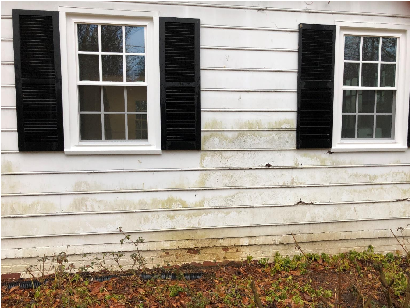
Figure 2: Deteriorated siding on addition
