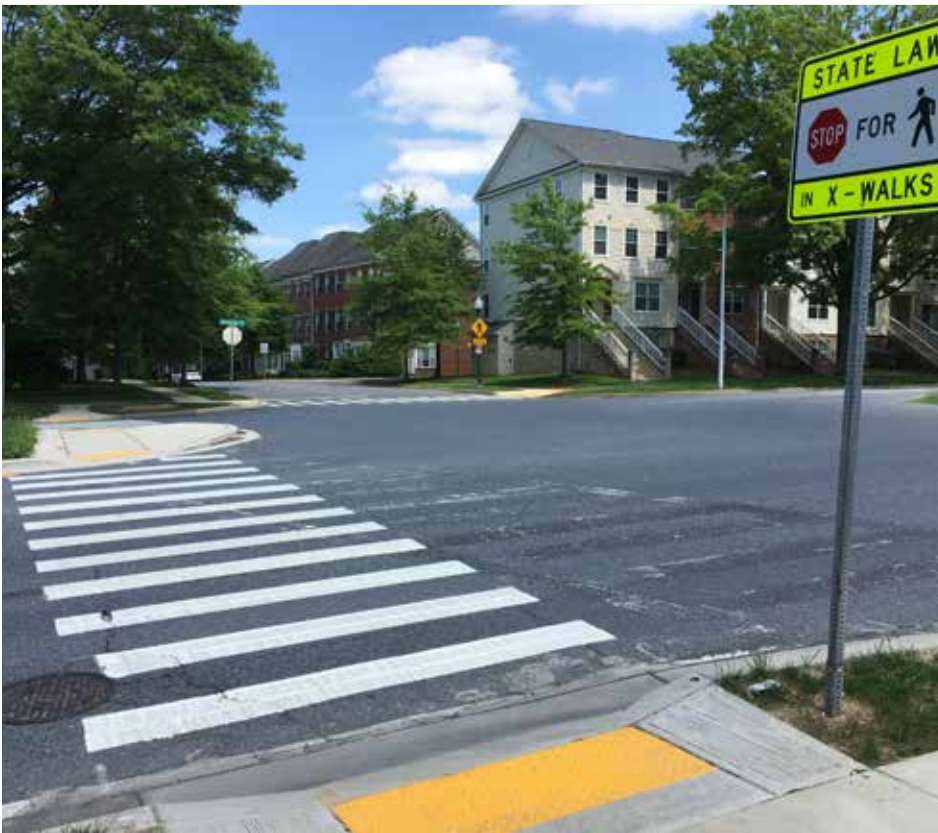
Figure 6-18. Street corner with two perpendicular curb ramps that align with crosswalks
