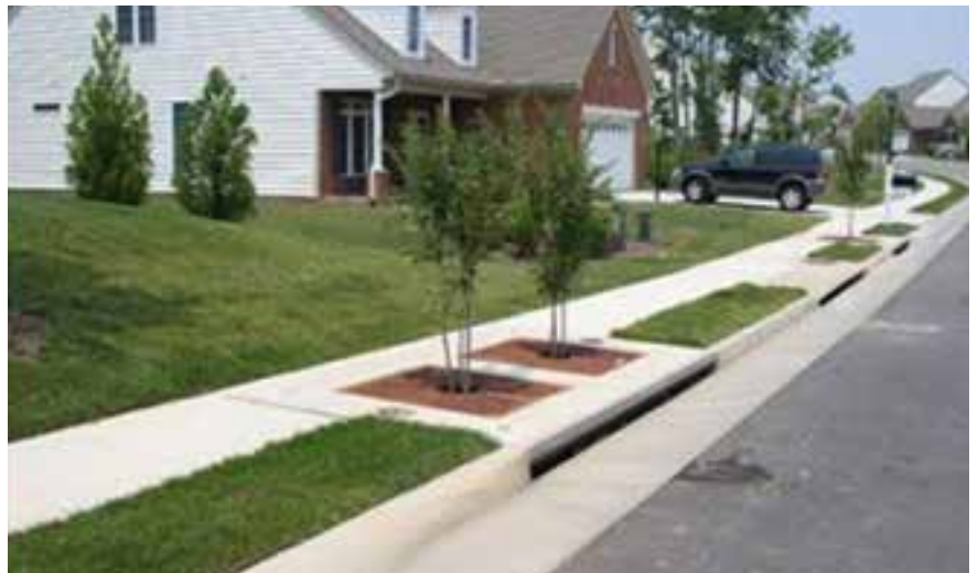
Figure 7-8. Examples of other green infrastructure BMPs (Source: Montgomery County Department of Environmental Protection)
