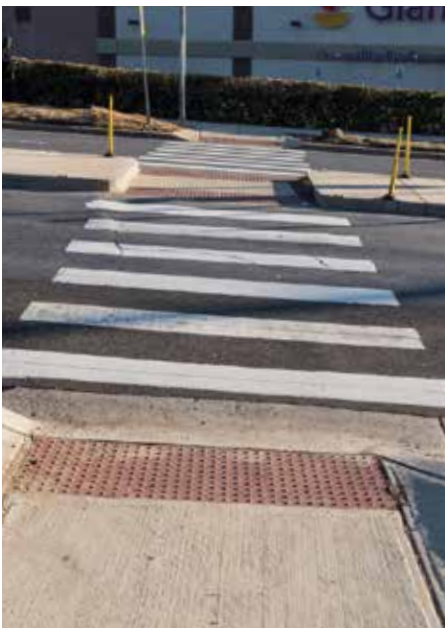
Figure 6-26. Example graphic and photo of a continental crosswalk
