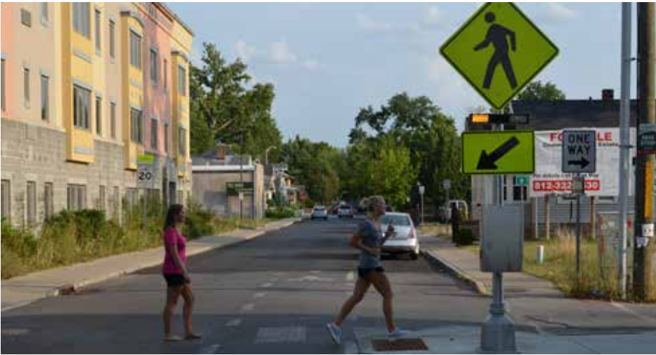
Figure 6-32. A Rectangular Rapid Flashing Beacon (RRFB)
