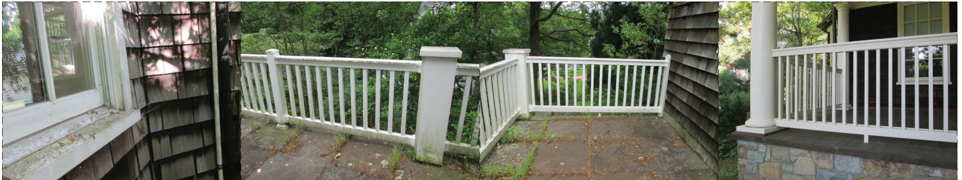
PHOTOS OF CURRENT 2ND FLOOR DECK RAILING WITH EXPOSED FASTENERS AS COMPARED TO MORE TRADITIONAL 1ST FLOOR PORCH RAILING
