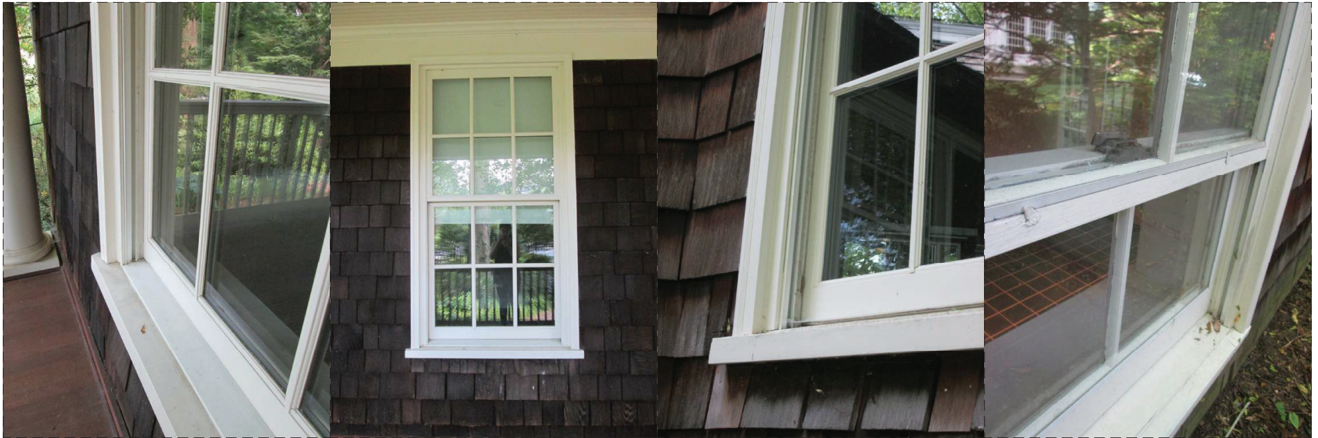
EXISTING WINDOW PHOTOS SHOWING PLASTIC JAMB LINERS, SPACER BARS AT SDL WINDOWS AND MODERN SASH LOCK HARDWARE
