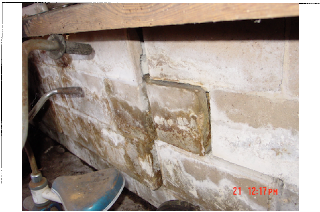
Detail: 40 Columbia Avenue - Garage interior detail, failed/buckled foundation.
