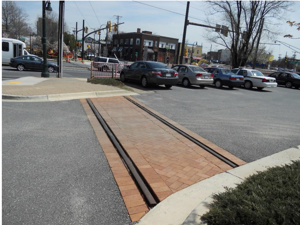
Photo 3 – Rails and Brick pavers installed at the entrance into the B&O Station Parking Lot prior to the construction of the Progress Place
