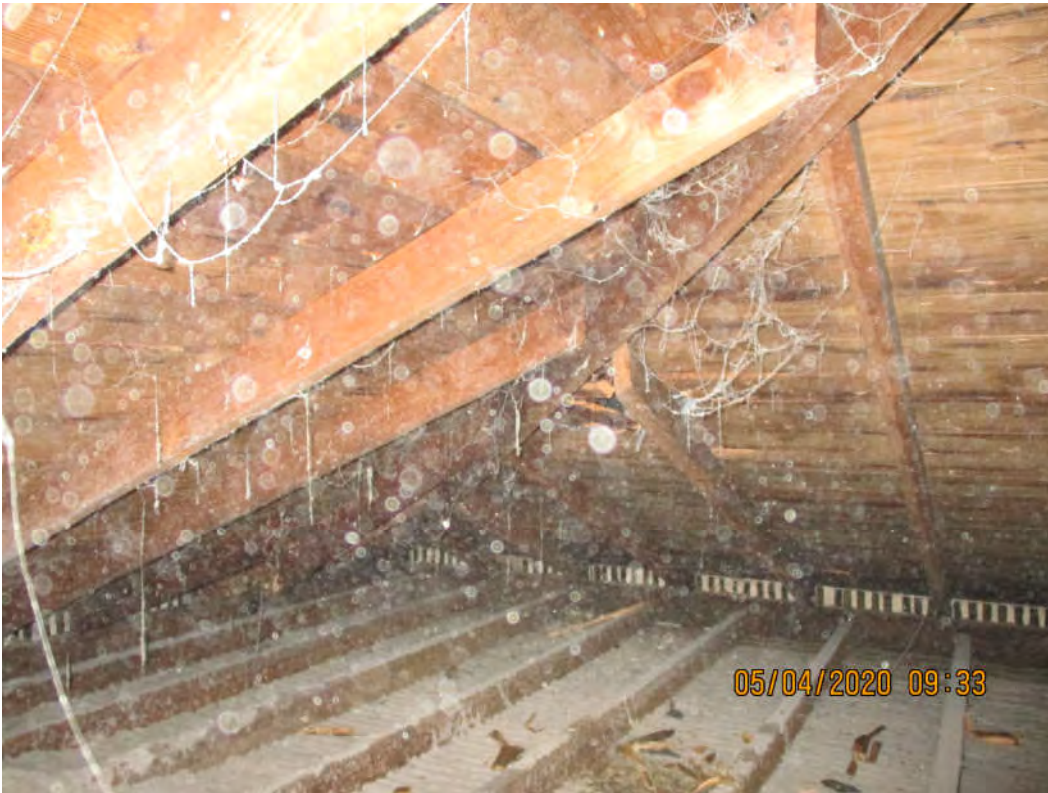
Figure 8. Broken/displaced hip rafters
