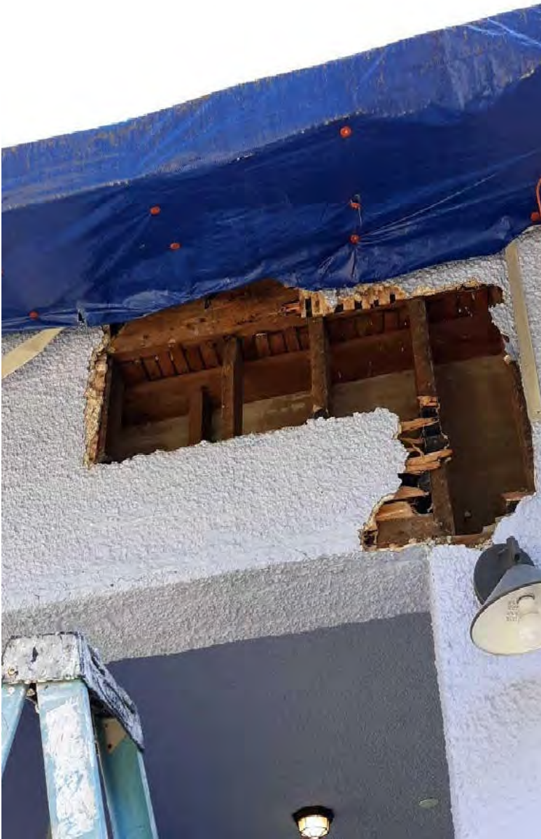
Figure 9. Hole opened up in stucco box over stairs
