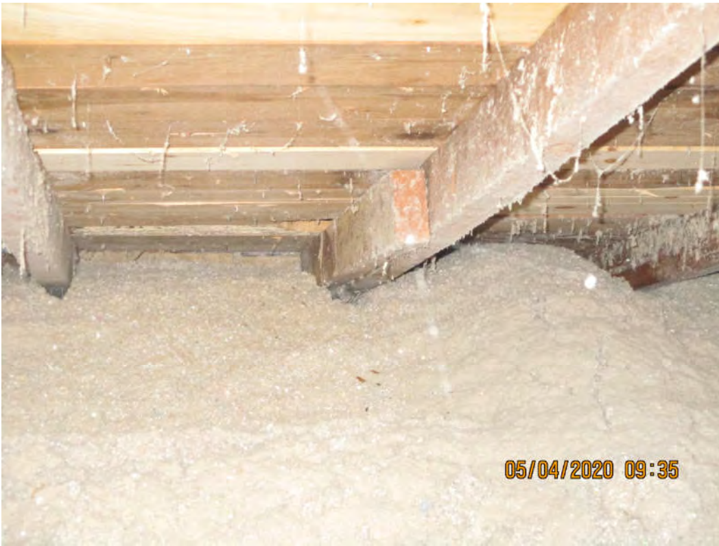
Figure 7. Broken/cracked common rafters
