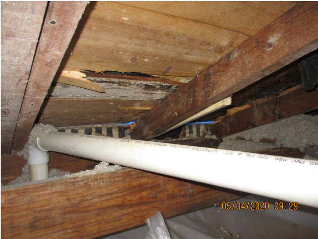
Figure 6. Broken/cracked common rafters
