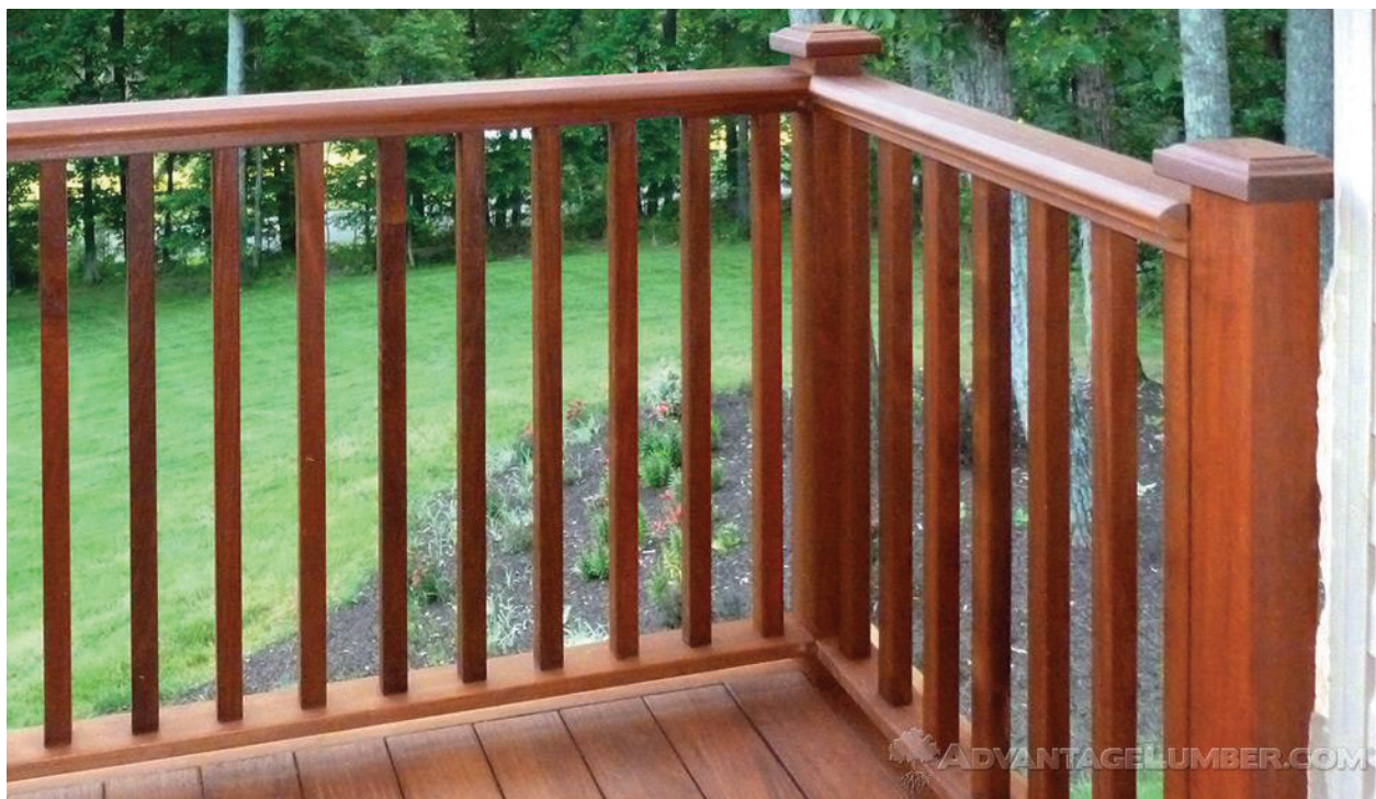
Figure 2: Example of a railing where the pickets are installed between the top and bottom rails.
