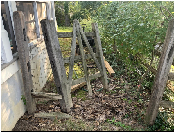
2. Existing fence - rot, failure, missing boards
