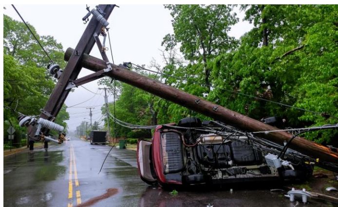
Figure 13: Storm damage in a residential neighborhood
