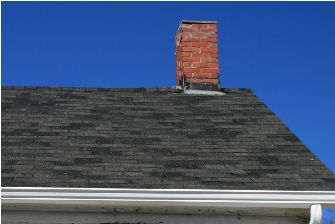
Photo 12 Close up view of existing 3-Tab shingles to be replaced like-in-kind. Photo by Ward Bucher | March 01, 2020
