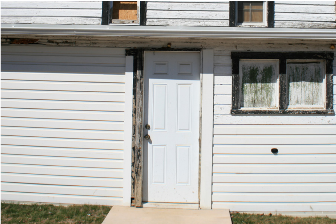
Photo 11 Existing door #104A to be enlarged on Side Facade (South Elevation). Existing dimensions are 6'-6" HT x 2'-6" WD Photo by Ward Bucher | March 01, 2020
