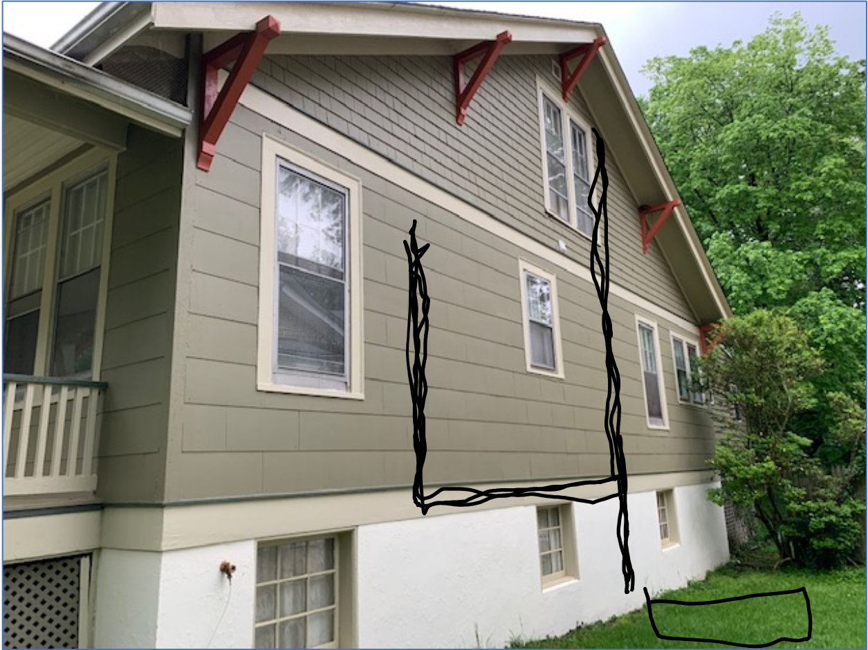
Detail: Photo showing the Eastern side of the house with approximate path of plumbing shown in black scribble pen. Box is approximate location of ground mount condenser unit.
