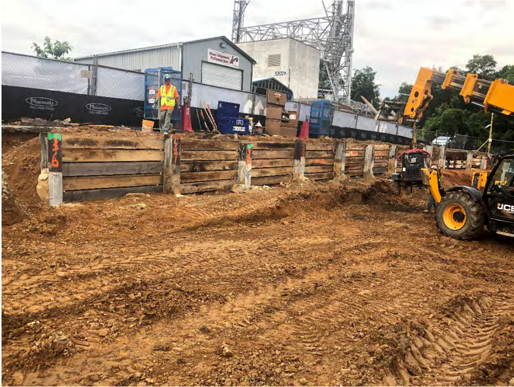
Figure 2: Installed Shoring; View to Southeast
