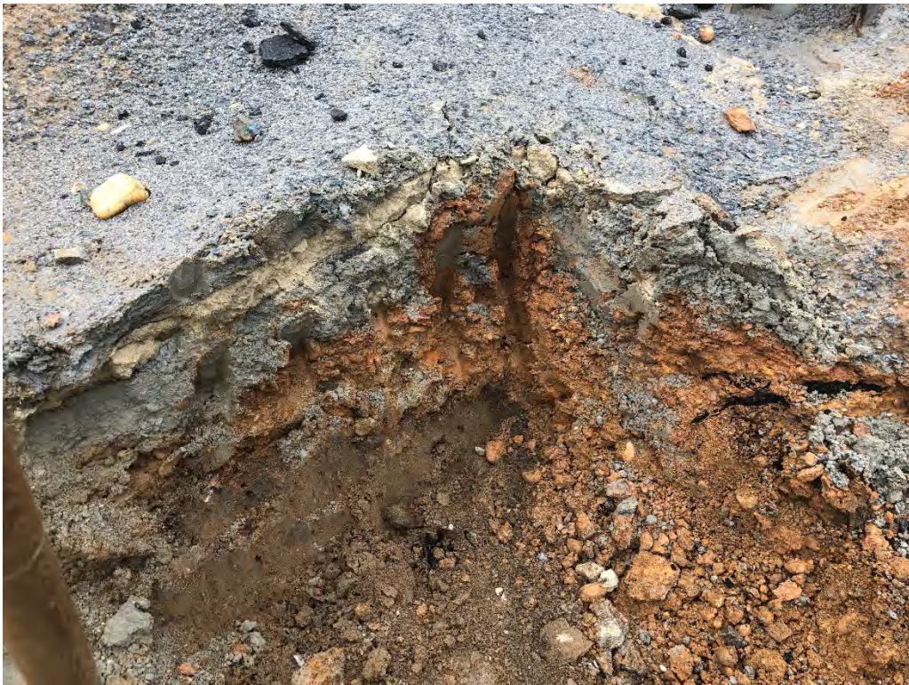
Figure 1: Fill Strata, View to Southeast
