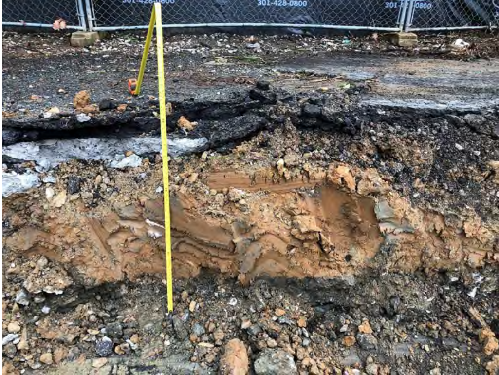
Figure 2: Excavation Profile; View to North
