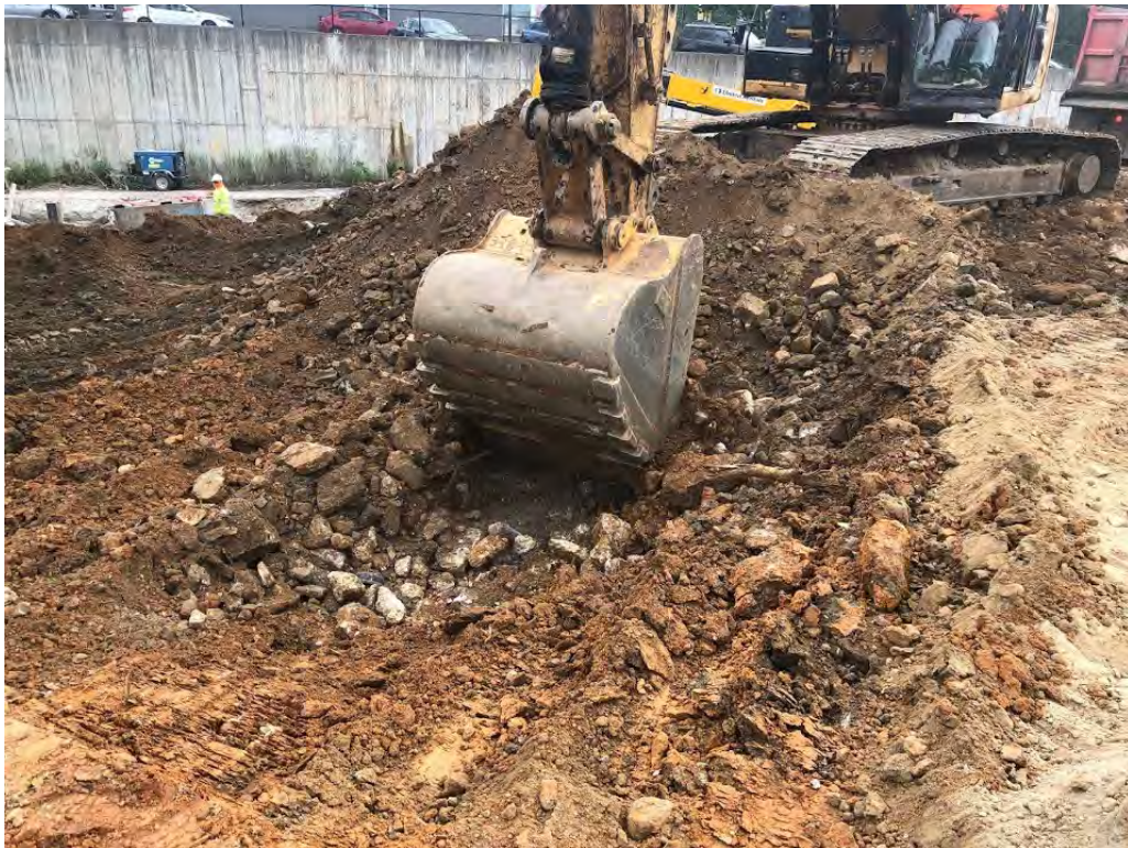
Figure 3: Rubble and Fill Soils, View to Northeast
