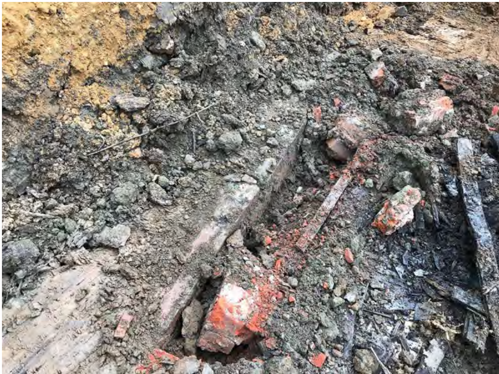
Figure 3: Remains of 20 th - Century Building, View to Northeast
