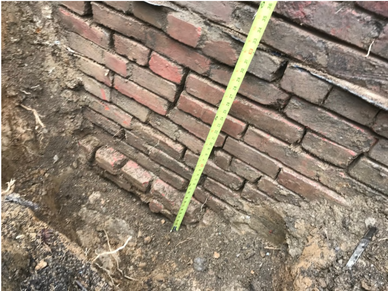
Sample foundation test pit showing deteriorated mortar and water infiltration areas.
