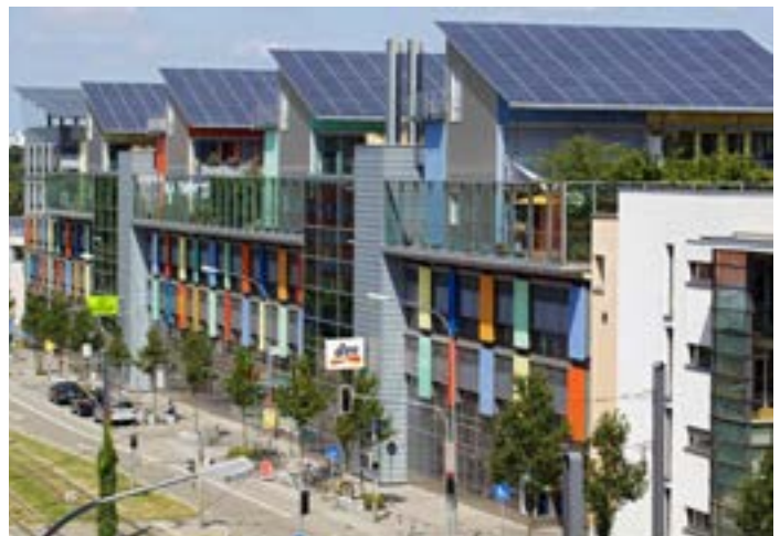
Rooftops oriented to maximize solar access.
