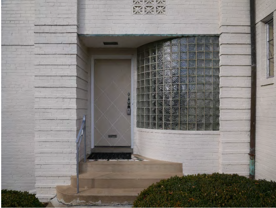
Figure 3: Detailed view of the front door on the east elevation.
