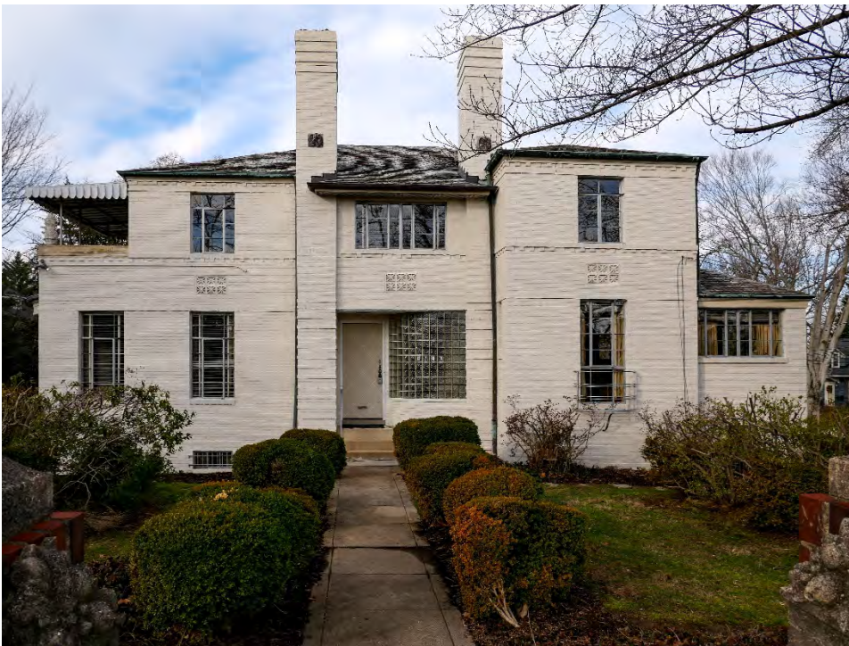
Figure 2: View of the east elevation (façade) looking west from the entrance gate.
