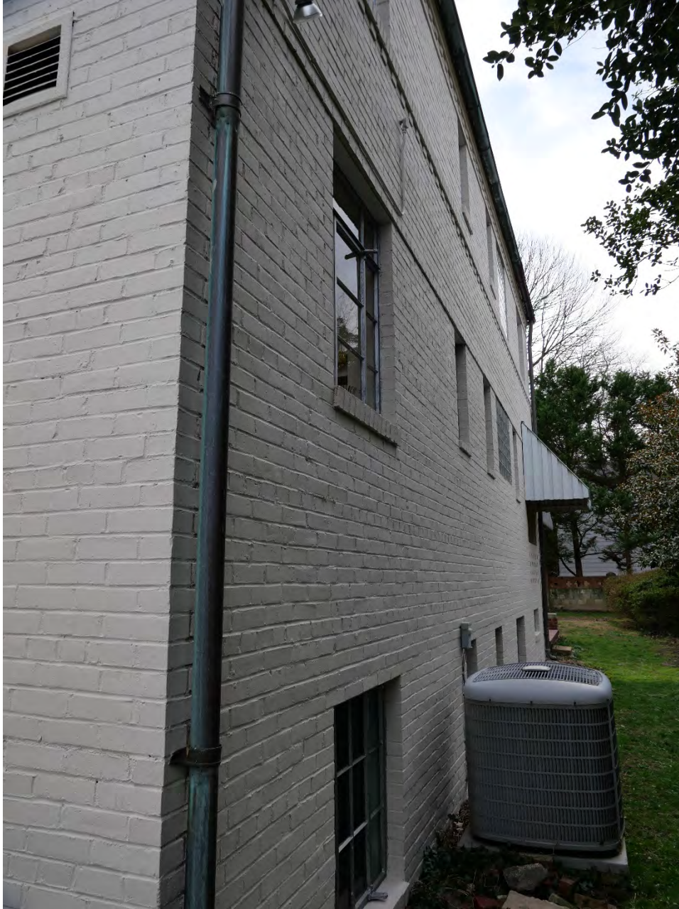
Figure 8: Partial view of the west (rear) elevation looking south.
