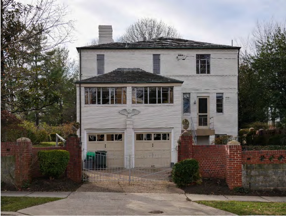
Figure 9: View of the north elevation looking south from Woodbine Street.
