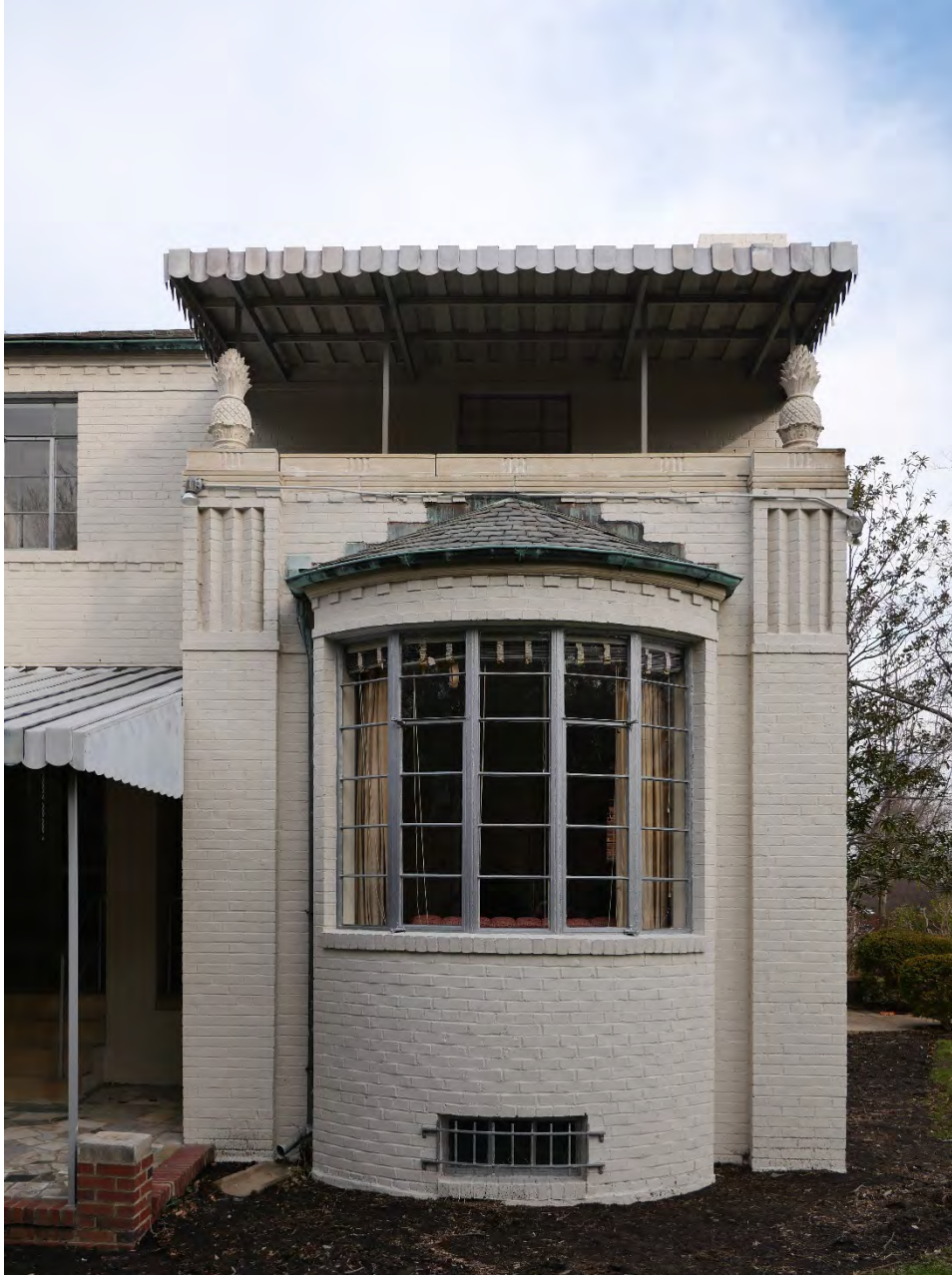
Figure 5: Detailed view of the bay window on the south elevation.
