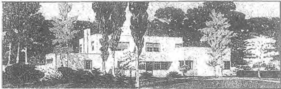
The first pre-fabricated motohome to be built in the Washington area is under construction on Brookside drive, in Kenwood, Chevy Chase, Md., for Lee D. Butler, prominent Washington automobile distributor. The house is built of prefabricated steel into which are set fireproof panels of compressed asbestos and cement, said to be indestructible. The house contains 12 rooms, 3 baths and a 2-car garage. A moto-unit, a mechanism no larger than a pantry, operates the air-conditioning, heating and hot water units. The above sketch is an artist's conception of what Mr. Butler's new home will look like when completed.
