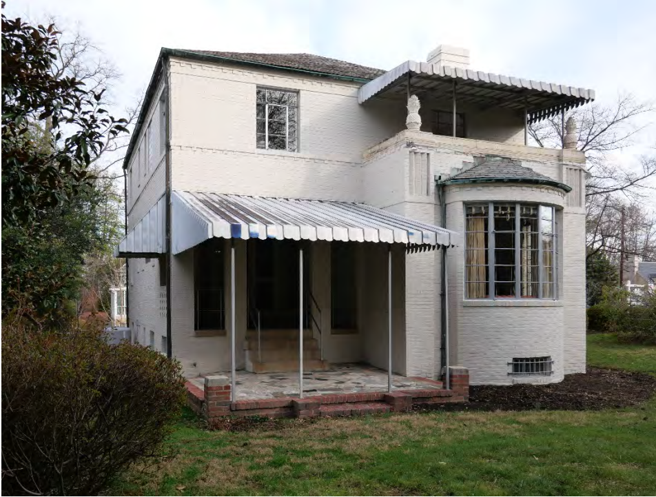
Figure 6: View of the south and west (rear) elevations looking north.
