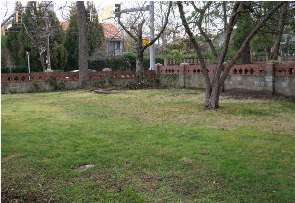
Figure 14: View of the front yard and brick and concrete block retaining wall looking east from the southern part of the property.
