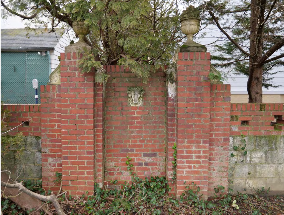
Figure 15: Detailed view of the southern section of the brick and concrete block retaining wall.
