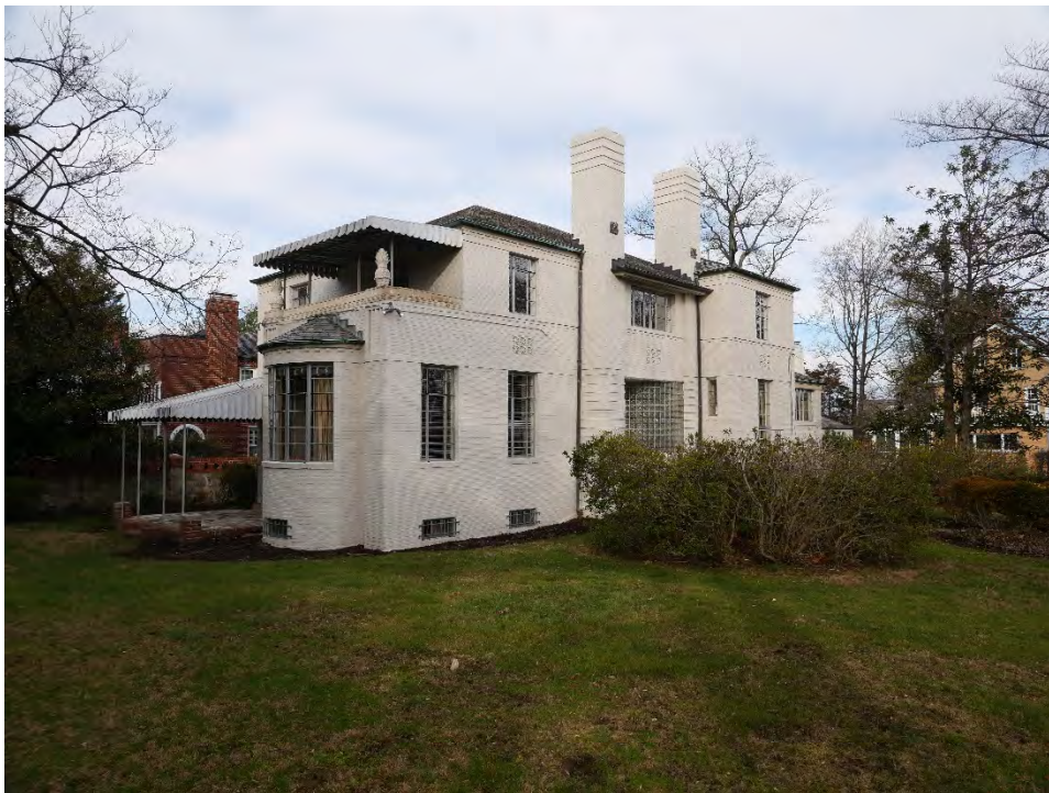
Figure 4: View of the south and east elevations looking northwest.
