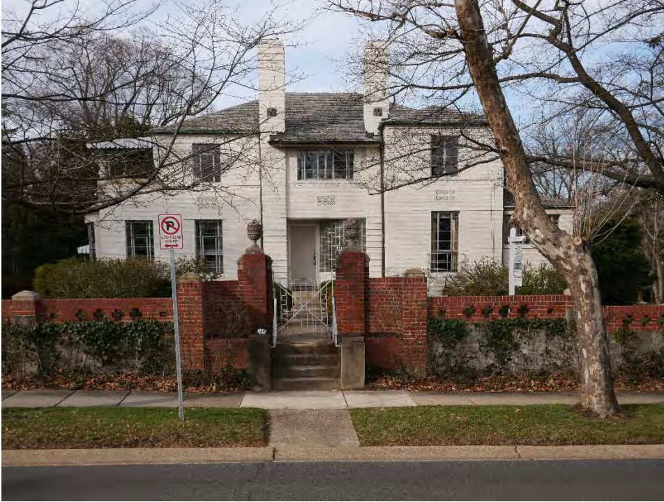
Figure 1: View of the east elevation (façade) looking west from Connecticut Avenue.
