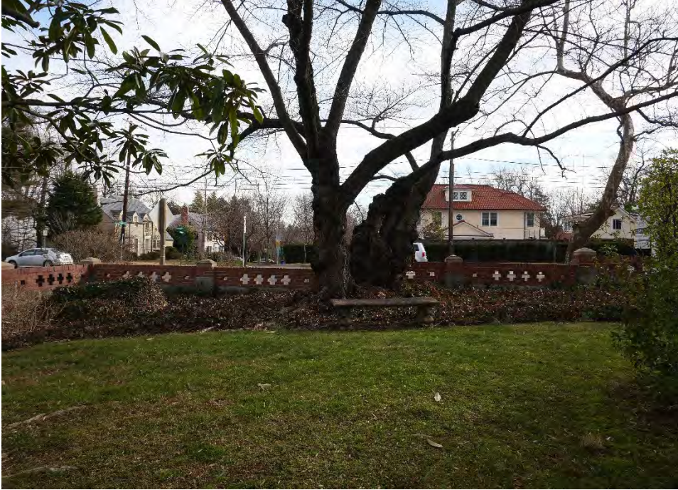
Figure 13: View of the front yard and brick and concrete block retaining wall looking east from the northern part of the property.
