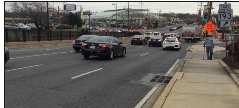
Figure 23. New Hampshire Avenue has no buffer between pedestrians on the sidewalk and the 35 mph roadway.
