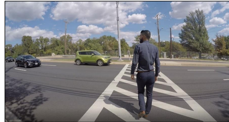
Figure 8. A two-stage, unsignalized crossing on 16th Street by 8600 Apartments (35 mph posted speed limit).
