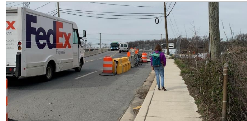
Figure 7. The sidewalk on the east side of Lyttonsville Place is being widened, but only on the northern segment as part of the bridge replacement. The southern half, pictured, remains narrow and without a buffer, despite connecting the station to the residential neighborhood south of the station.
