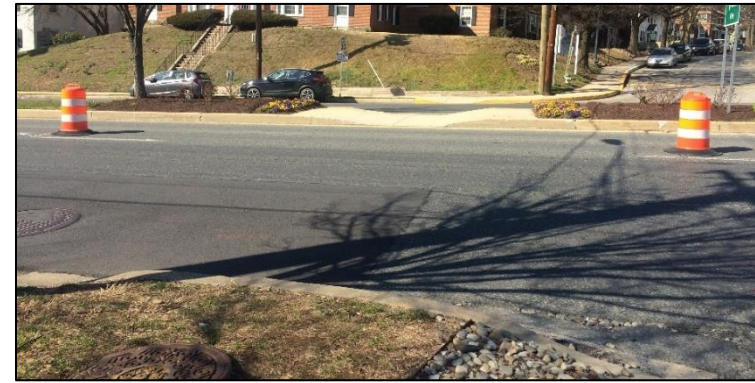
Figure 10. This crossing at Draper Lane and Colesville Road is missing a curb cut on the eastern side (as well as a crosswalk) and is the only crossing of Colesville Road between East-West Highway and 16th Street.
