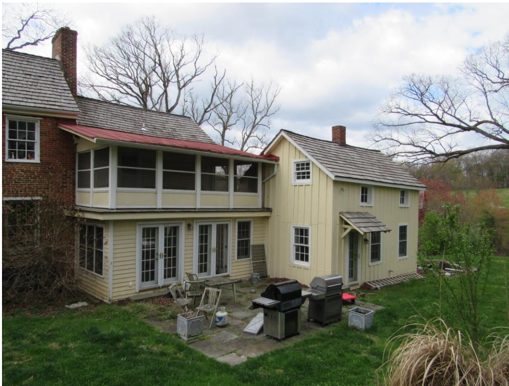
Fig. 4: North view, showing the previously enclosed porch, which connects the summer kitchen to the main house.
