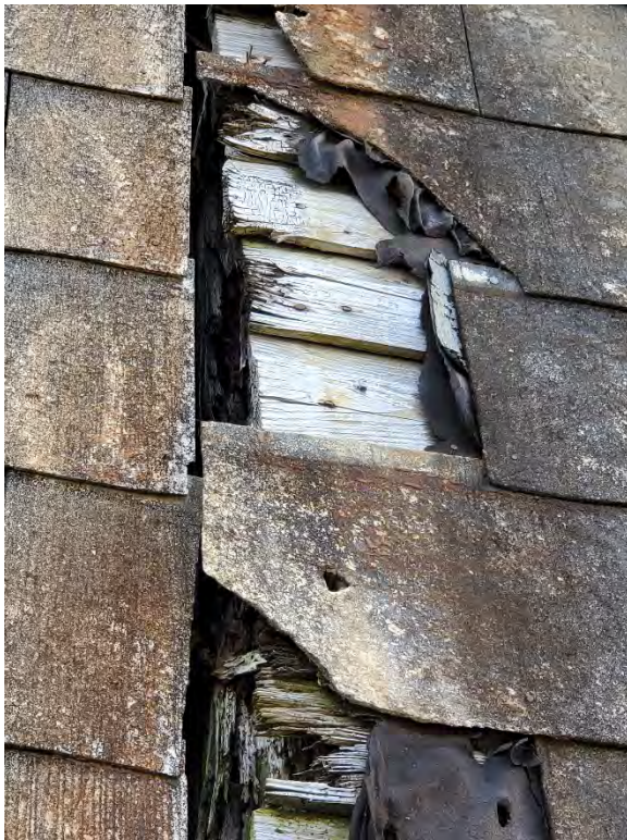
Figure 12: Detailed view of the exposed wood siding.
