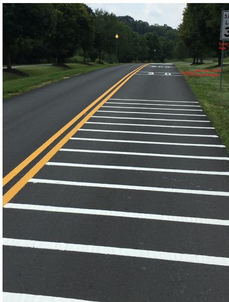
Figure 9-11. Example of optical speed bars
