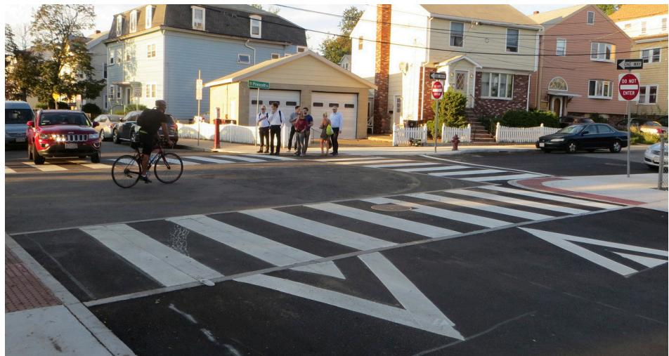
Figure 6-33. Image of a raised intersection
