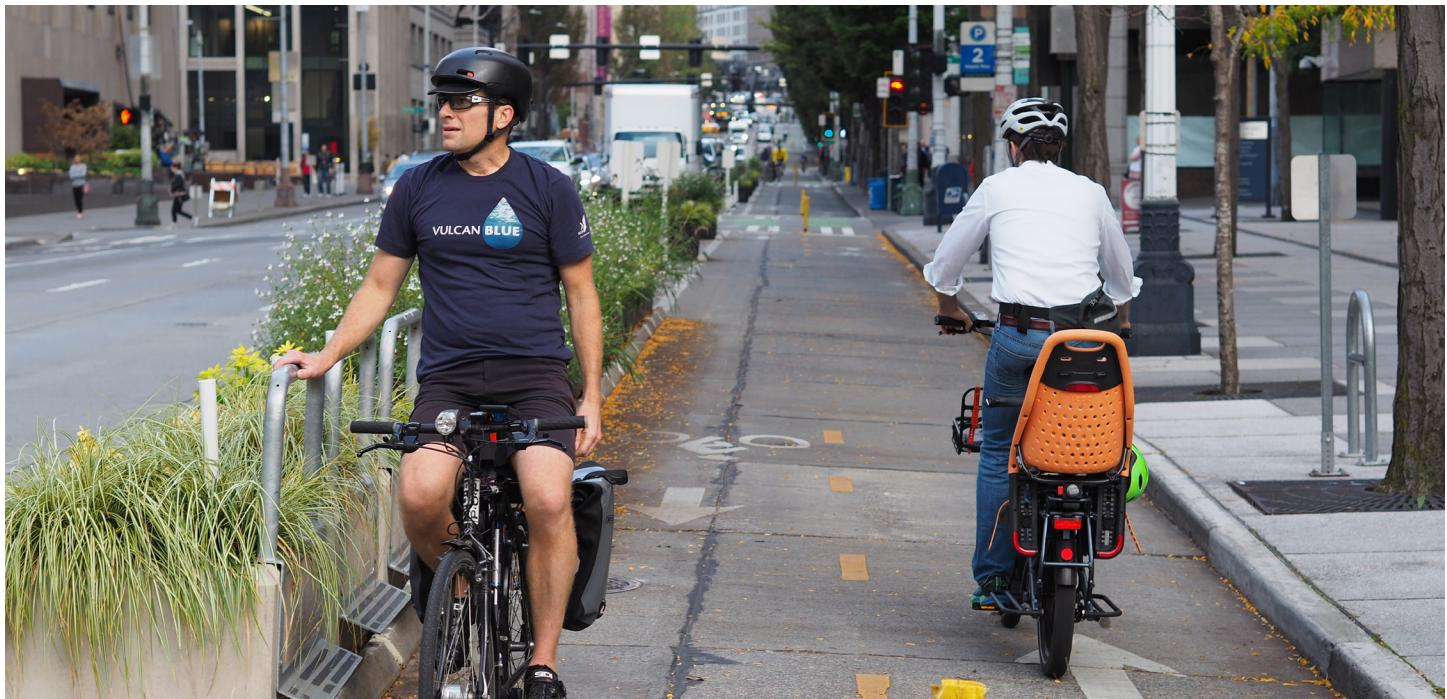
Figure 8-23: Example of bicycle lean rails and foot rests
