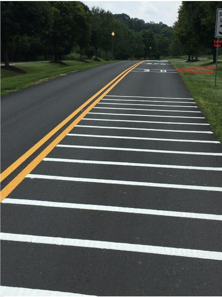
Figure 9-11. Example of optical speed bars
