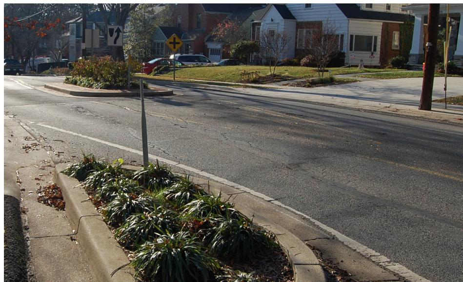
Figure 9-8: Horizontal traffic calming treatment
