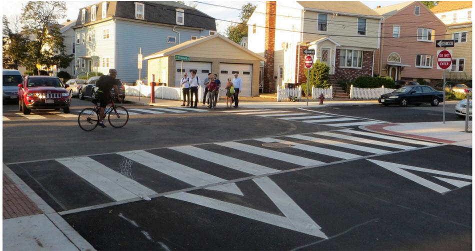
Figure 6-33. Image of a raised intersection
