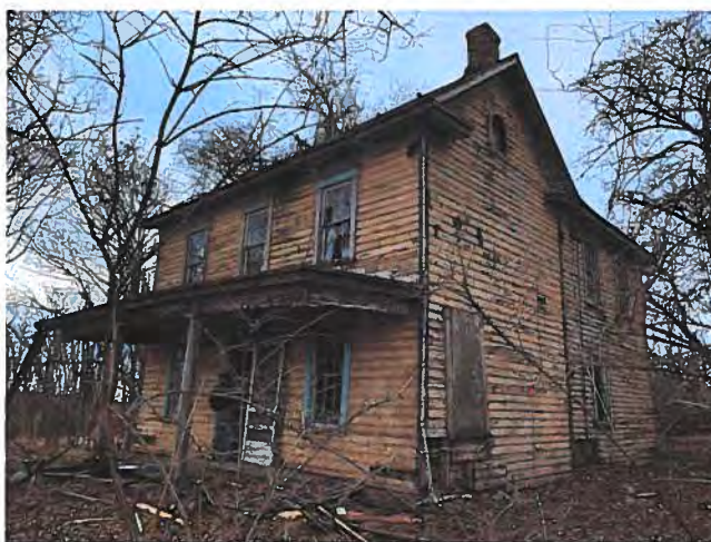
Fig. 2: West (front) and North sides. Note patches in siding below window indicating former door with stoop. 2020-01-02
