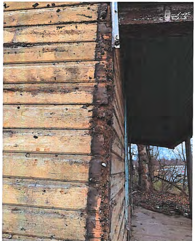
Fig. 8: Typical corner detail throughout showing paint line from removed corner board, insect and fungal damage. 2020-01-02
