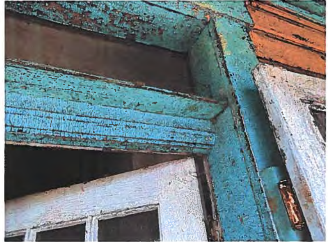
Fig. 10: Front door transom bar (Door head matches adjacent windows.) 2020-01-02
