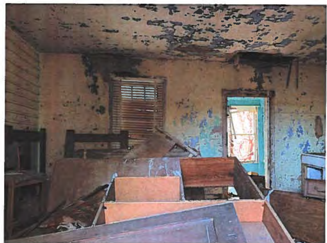
Fig. 16: East Room in Rear L, looking south. Note exterior siding on wall to Main House on left. 2020-01-02
