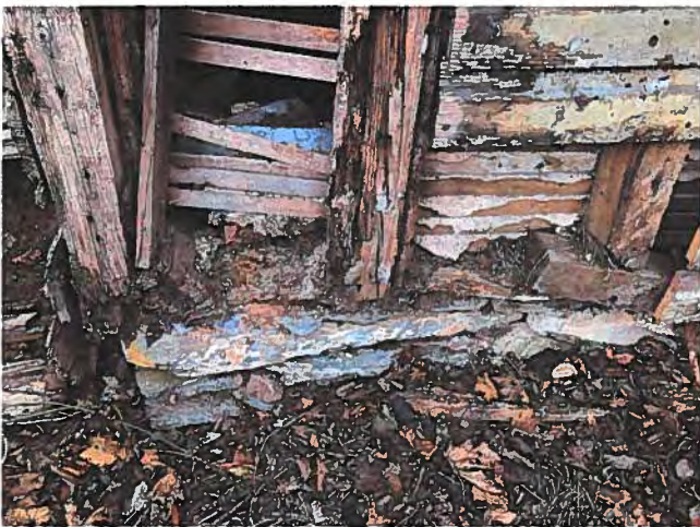
Fig. 11: Looking into opening at north west corner showing deteriorated/non-existent sill plate (front wall sill plate and front porch on left), studs, joists, joists laid directly on earth. 2020-01-02
