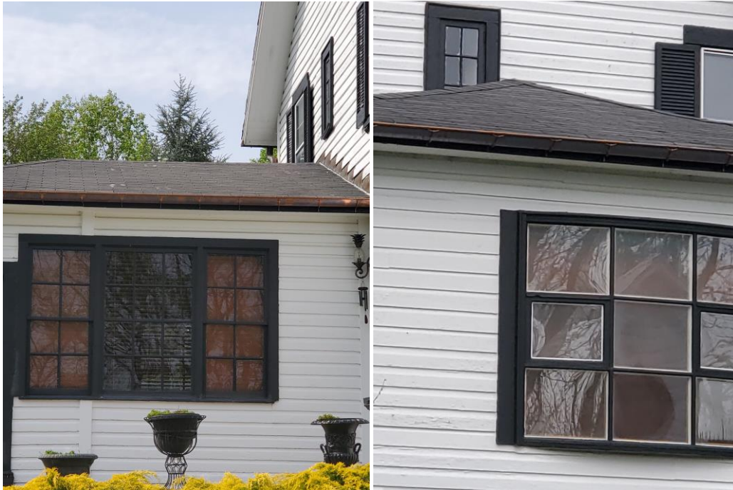
Figure 1: Views of Existing 3-Tab Asphalt Shingle Roof
