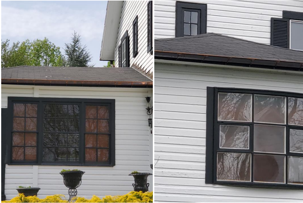
Figure 1: Views of Existing 3-Tab Asphalt Shingle Roof
