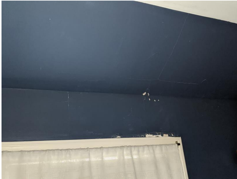
Figure 3. Water damage below low-sloping shed dormer roof
