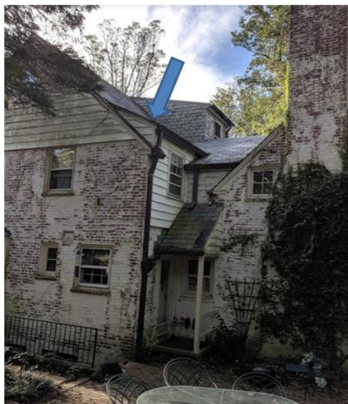
Figure 2. Converging roof sections above side porch
