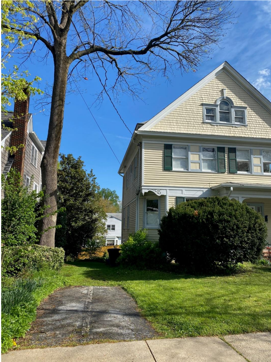
3713 Underwood Street – Non-original deteriorated asphalt driveway pad
