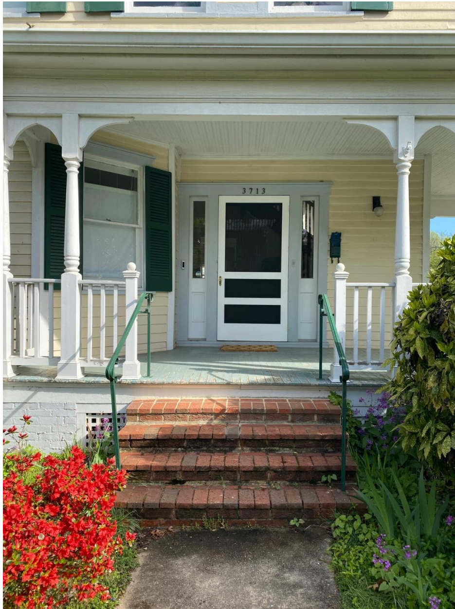
3713 Underwood Street - Non-original deteriorated brick front porch steps
