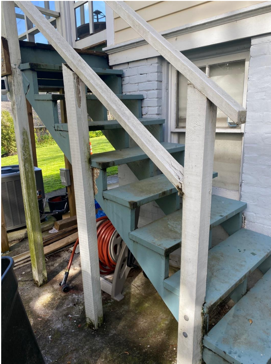
3713 Underwood Street – Deteriorated back porch stair
