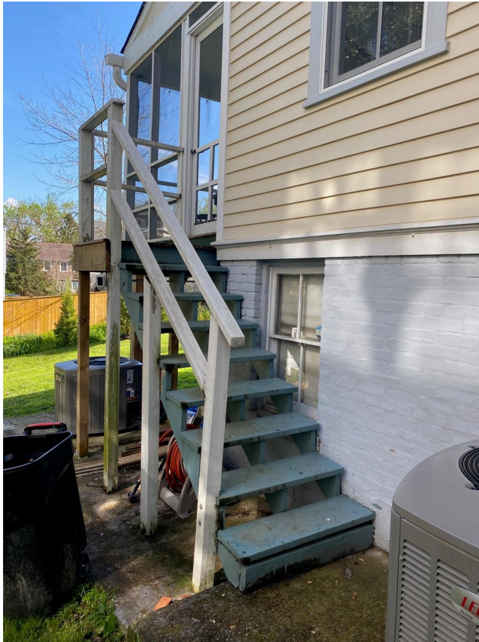
3713 Underwood Street – Deteriorated back porch stair
