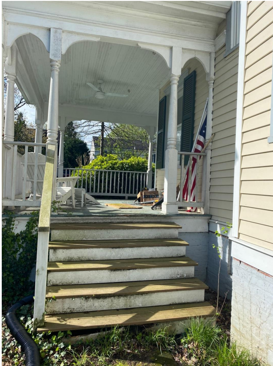
3713 Underwood Street – Non-original deteriorated front porch side stair
