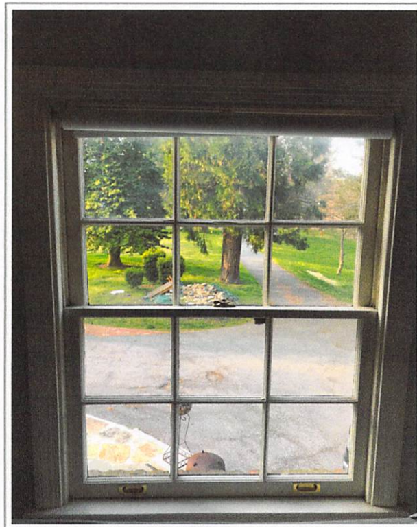
Detail picture of interior of double hung window.
