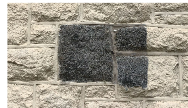
SAMPLE OF PAINT REMOVAL FROM EXISTING STONE
