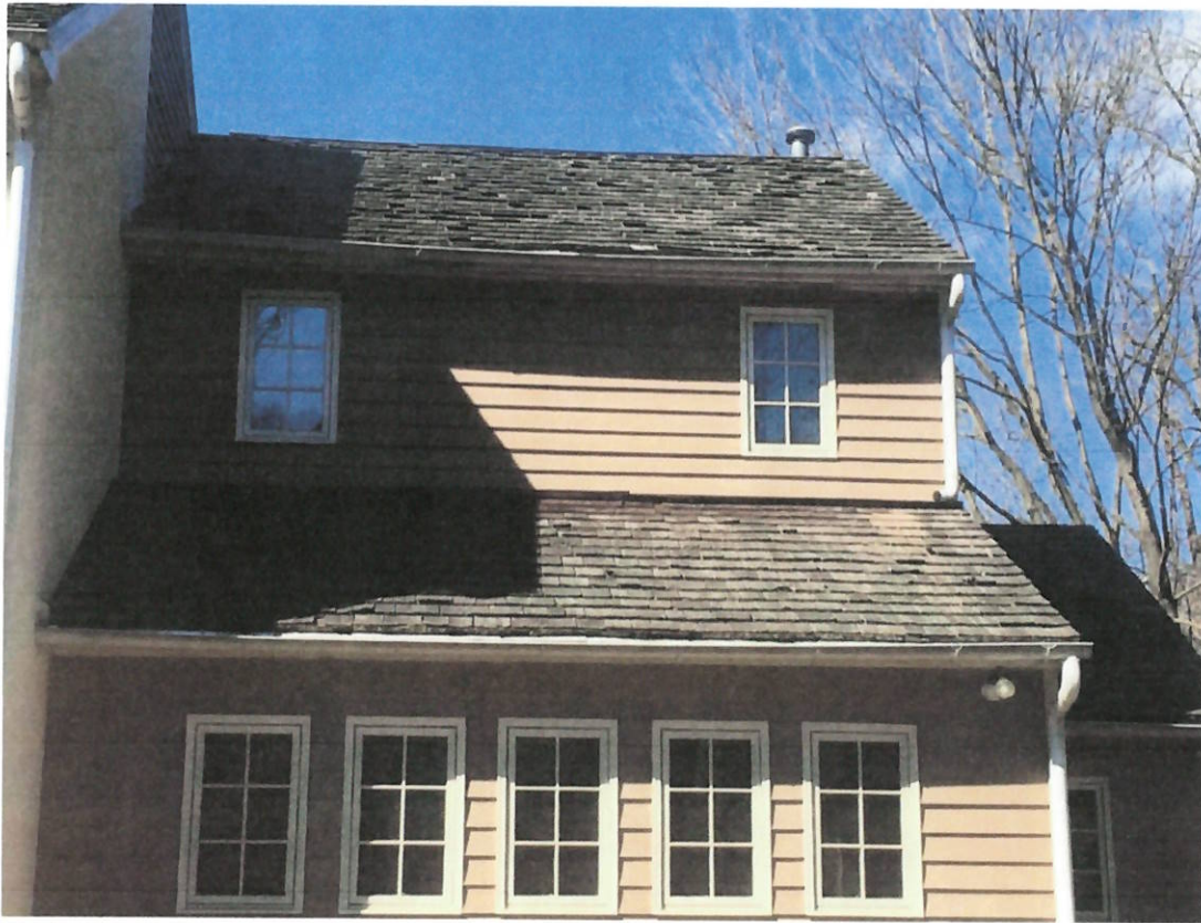
Damaged Shingles 1
