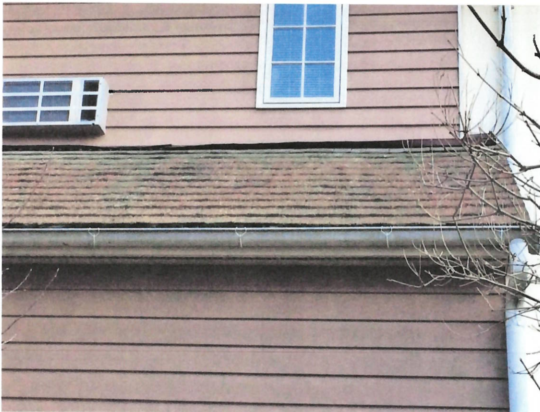
Damaged Flashing – Moss on Shingles
