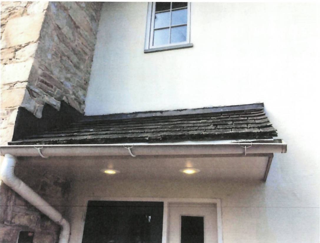
Damaged Shingles – Damaged Gutter 2
