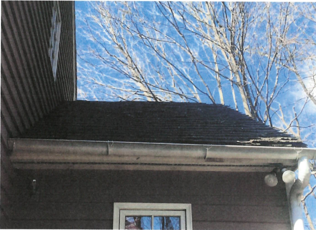
Damaged Shingles – Damaged Gutter 1
