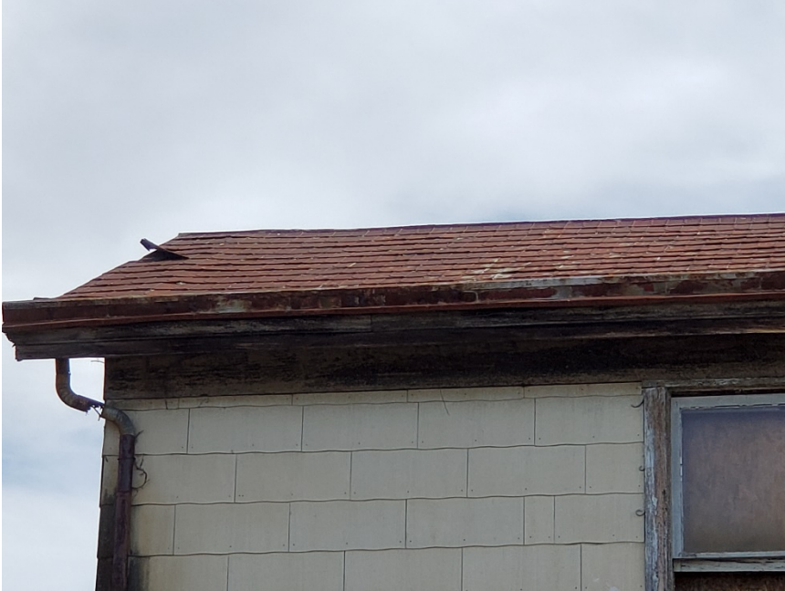
Figure 13: Detailed view of the stamped tin shingle roof on the two-story store.
