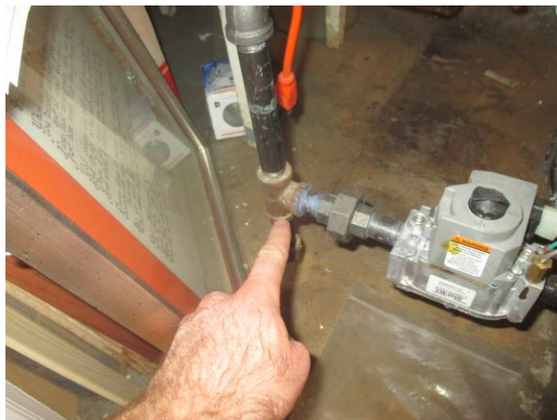
Gas leak detected near water heater
