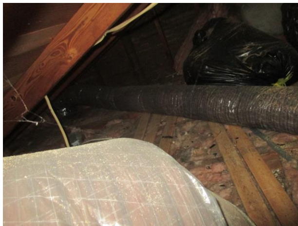
Current main attic insulation
