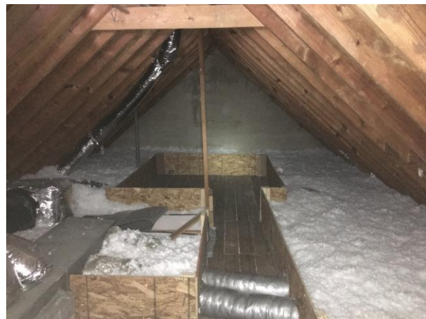
Well insulated R-49 attic with damming
