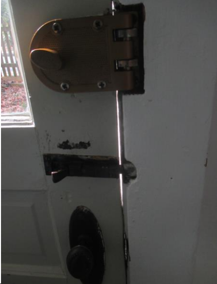
Current basement door weather-stripping
