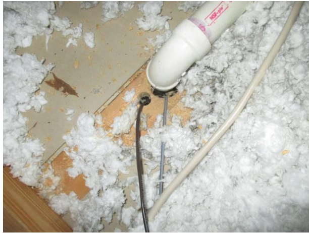
Common plumbing and wiring penetration
