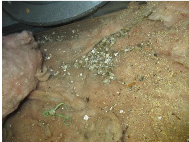
Potential vermiculite with asbestos
