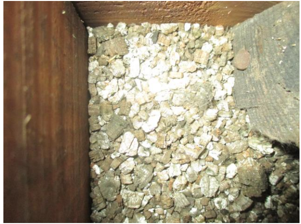
Vermiculite under fiberglass batts
