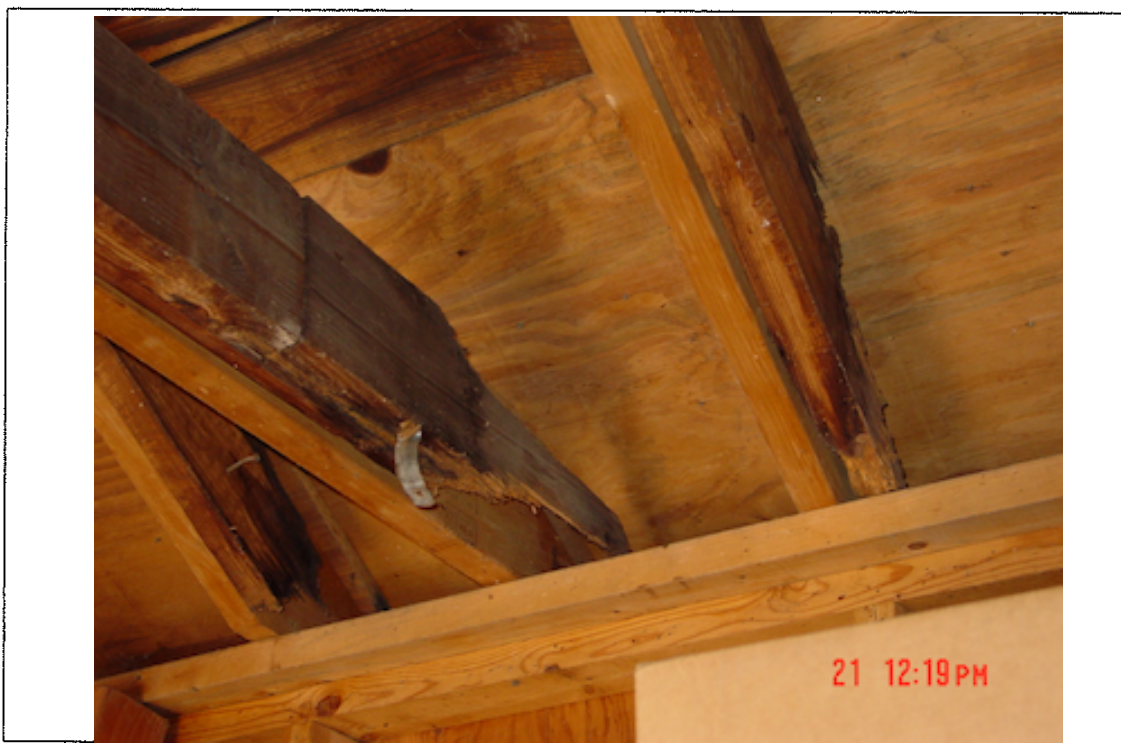
Detail: 40 Columbia Ave. - Garage interior detail, termite damage at rafters.
