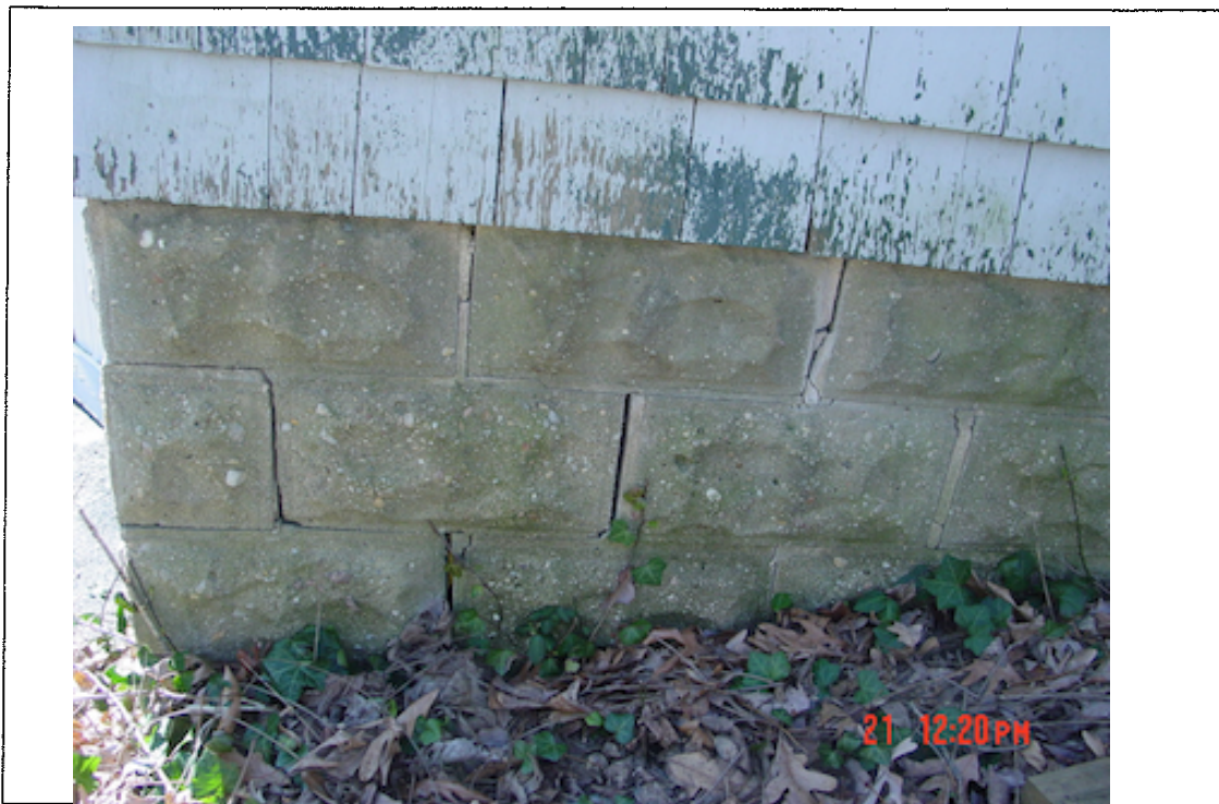
Detail: 40 Columbia Avenue - Garage exterior detail, failing foundation
