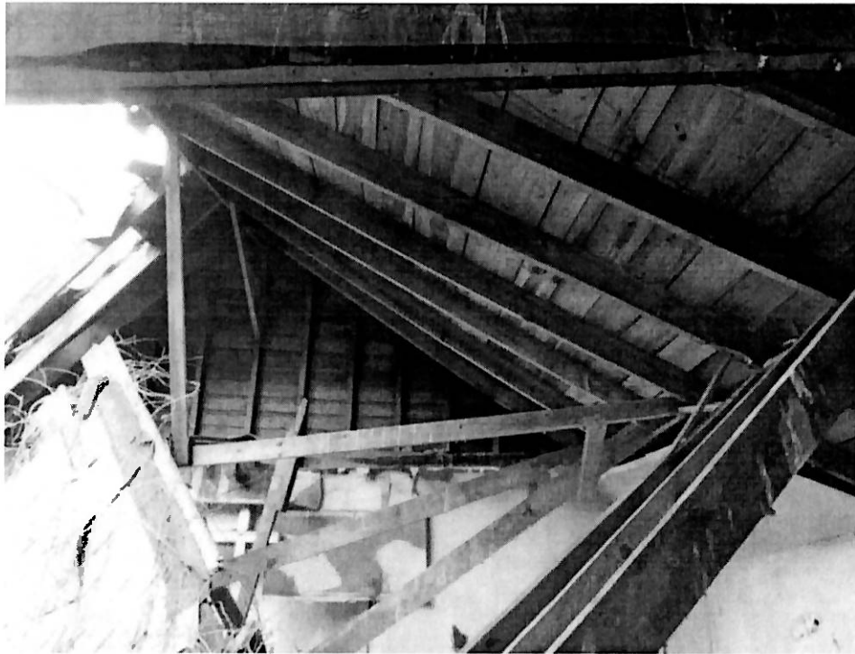
Photo No. 13: View collapsed roof framing along the west end of the structure. Note that wall and roof framing consists of 1" thick wood boards of various widths attached to solid sawn rafters or studs.
