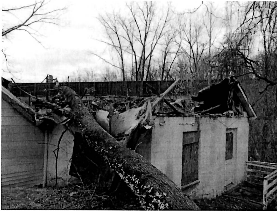
Photo No. 8: View of the southwest portion of the structure (see from the northwest) which has been impacted by a collapsed tree (purportedly in 2007).
