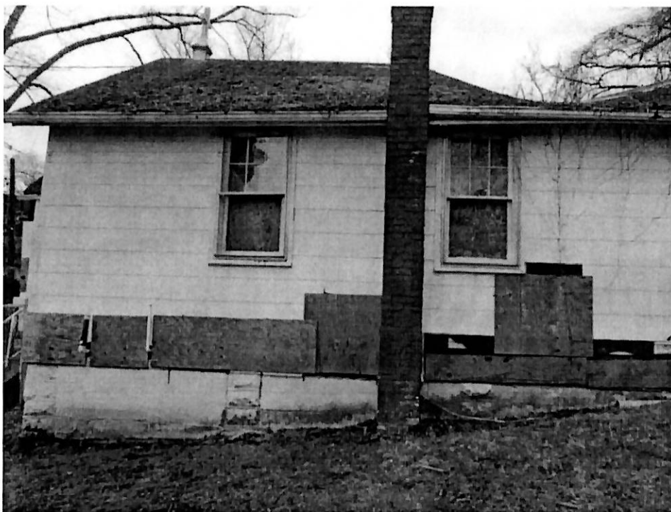
Photo No. 6: Partial view of the front half of the north elevation showing boarded wall openings and windows, extreme moss growth on the intact portion of the roof, as well as the collapsed section of the roof (right side).
