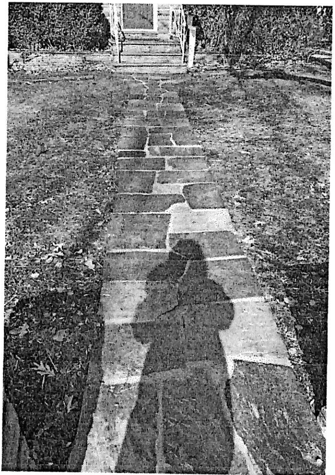
EXAMPLE: NEW FLAGSTONE ON CONCRETE FRONT WALK
