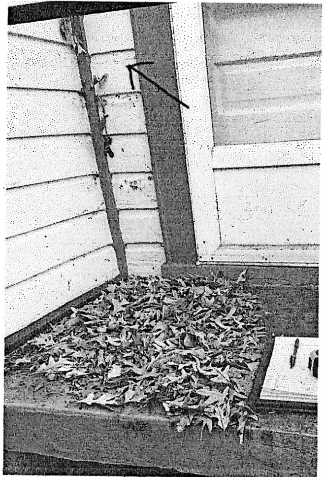
REAR ADDITION @ MAIN HOUSE SHOWING NON-ALIGNMENT OF SIDING
