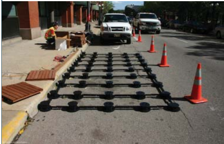
Completed bracing, Anchor to curb and road base.
