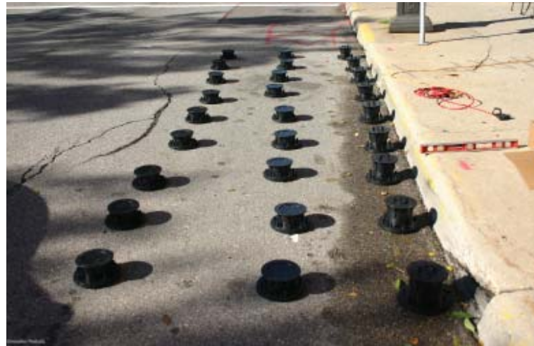
Set pedestals roughly 2 feet apart.
