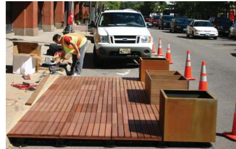
Install fascia boards, planters, & railing.
