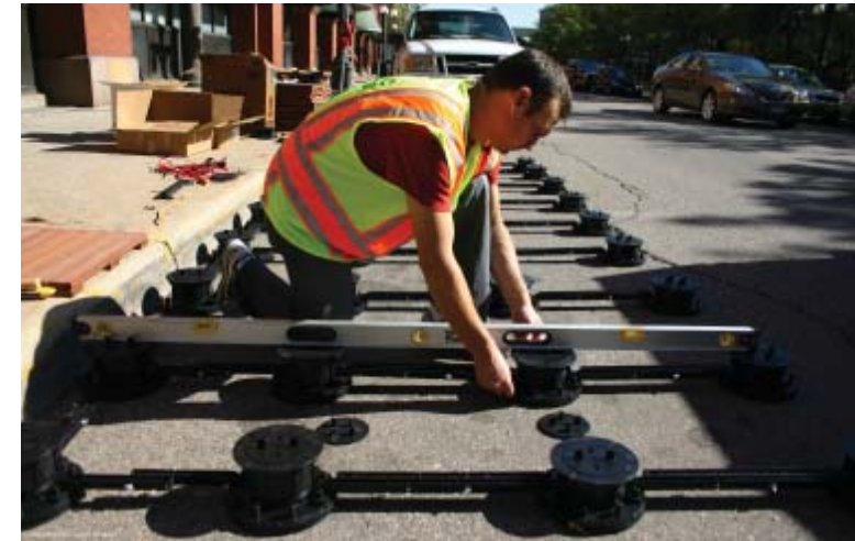
Level with Versadjust pedestal slope compensator and install bracing.
