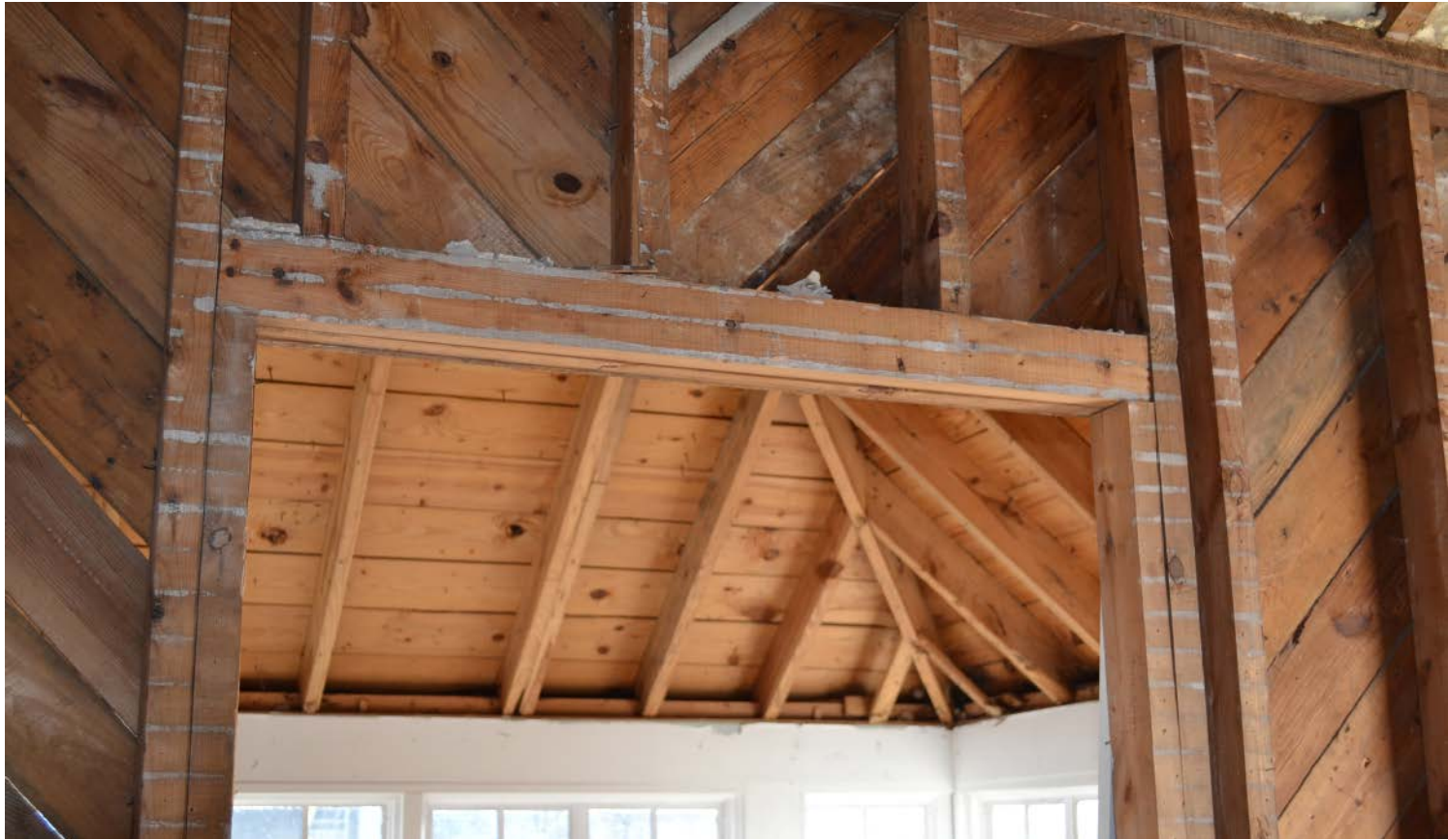
7. Study Entrance showing framing transition
