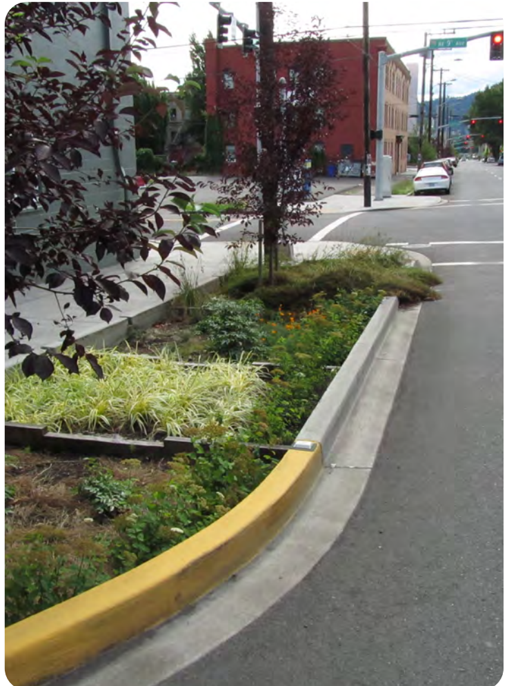
Reflective paint on curbs can help drivers see curb extensions and stormwater facilities along the road, avoiding collisions and damage.
