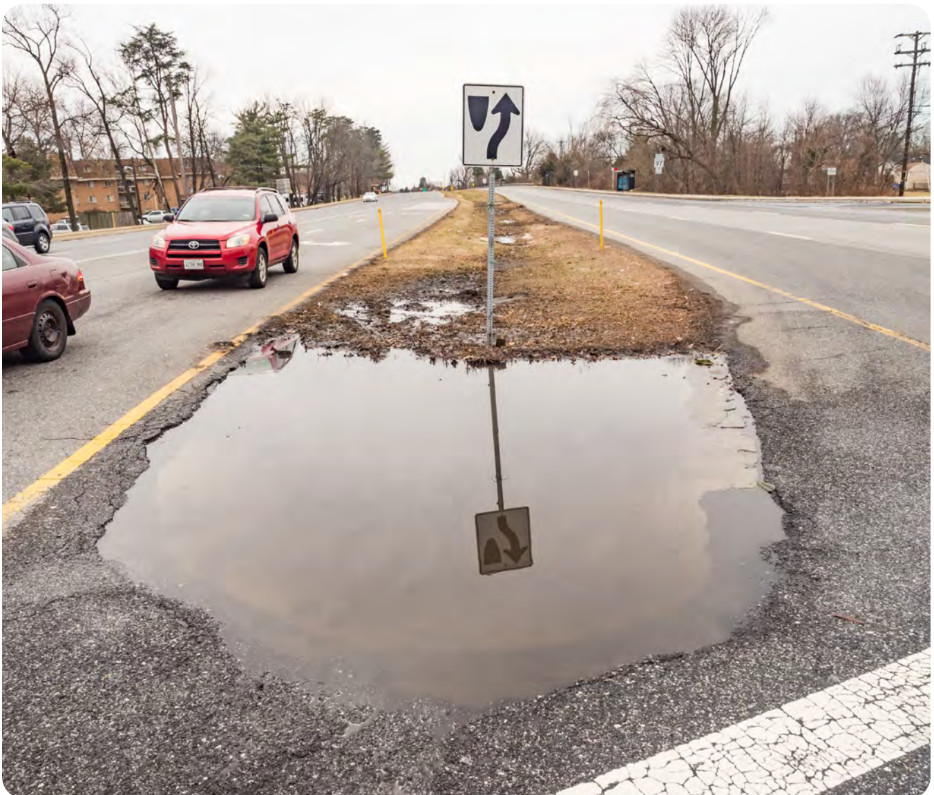
The median at Georgia Avenue and Bel Pre Road is typical of medians in the Aspen Hill area: they are not protected and may present barriers to people with mobility devices, strollers, and low or no vision. Refuge islands provide a safe space for people to rest or wait while crossing the roadway and may also be used for stormwater management.
