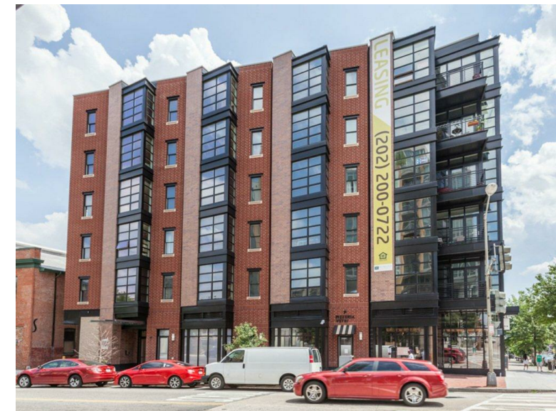
Articulated Facade to give direction and verticality
