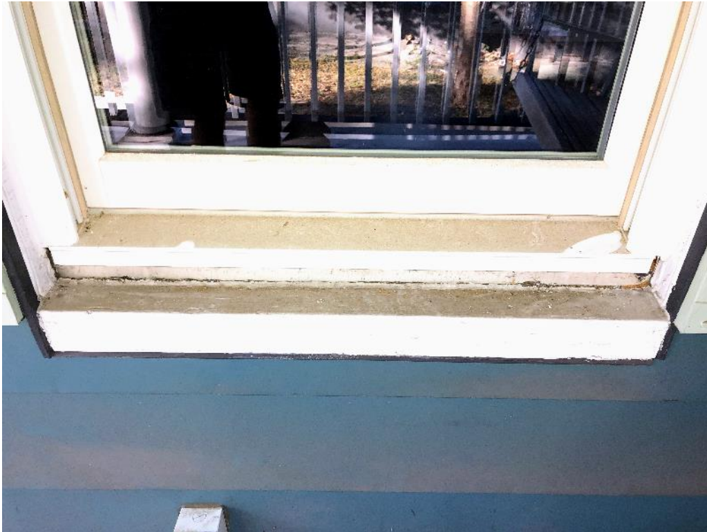
Damaged window sill that was previously wrapped in aluminum
