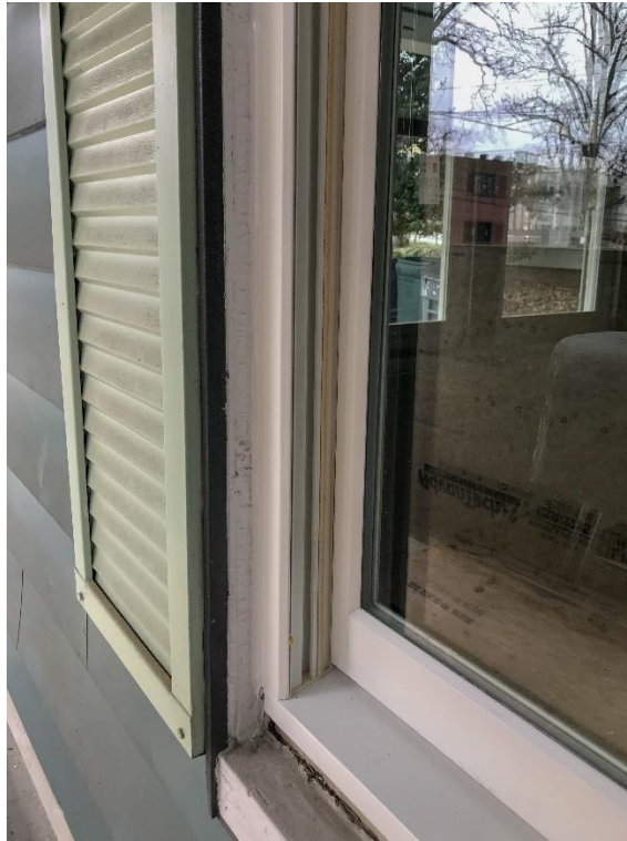
Figure 2: Detail of the exposed jamb liner.
