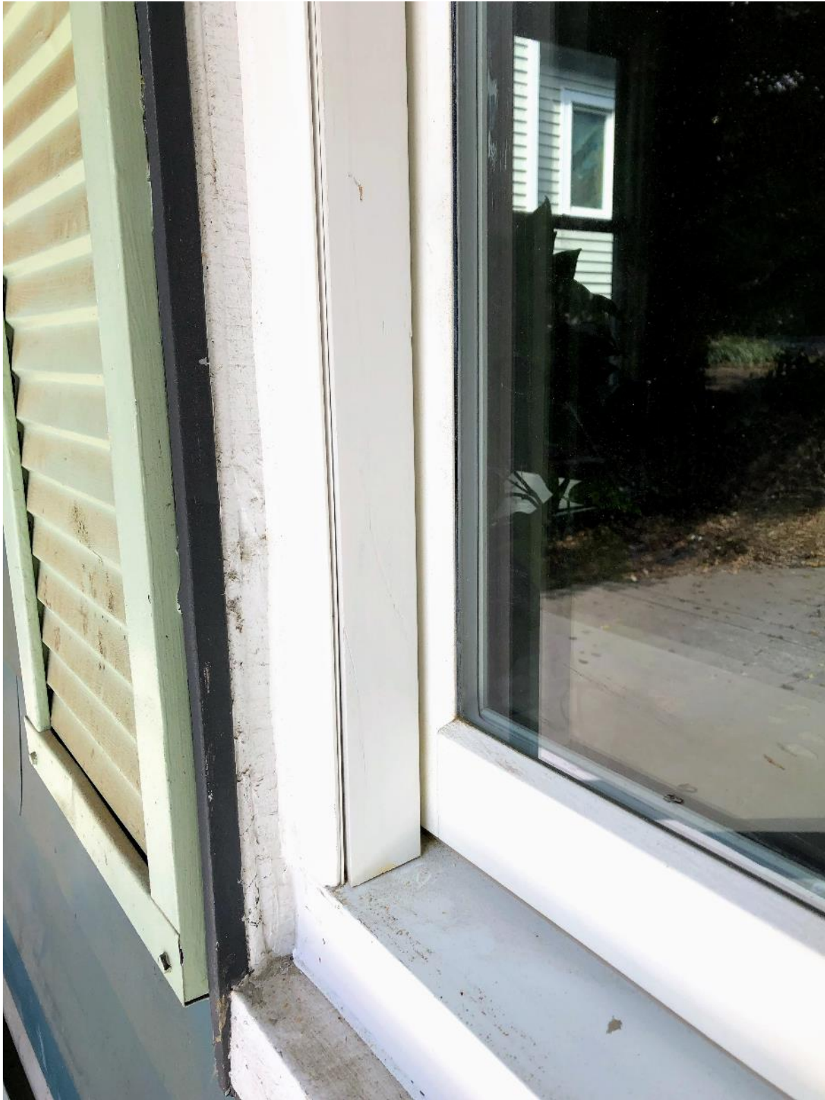
Close-up view of trim piece covering jamb liner
