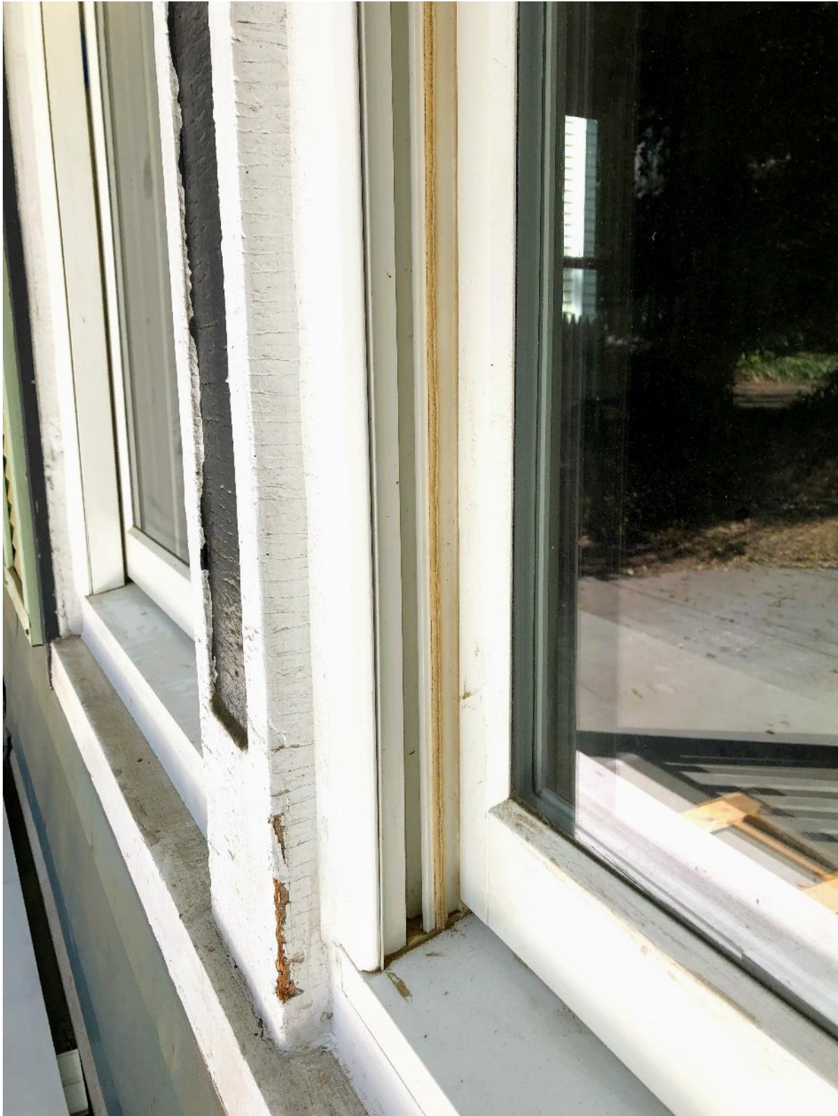
Window with wood jamb liner cover next to window with exposed jamb liner
