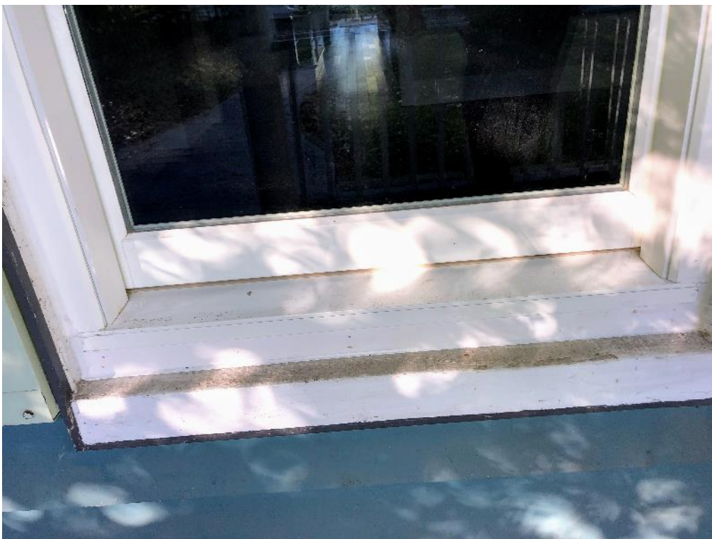
Mockup of new window sill constructed of solid wood
