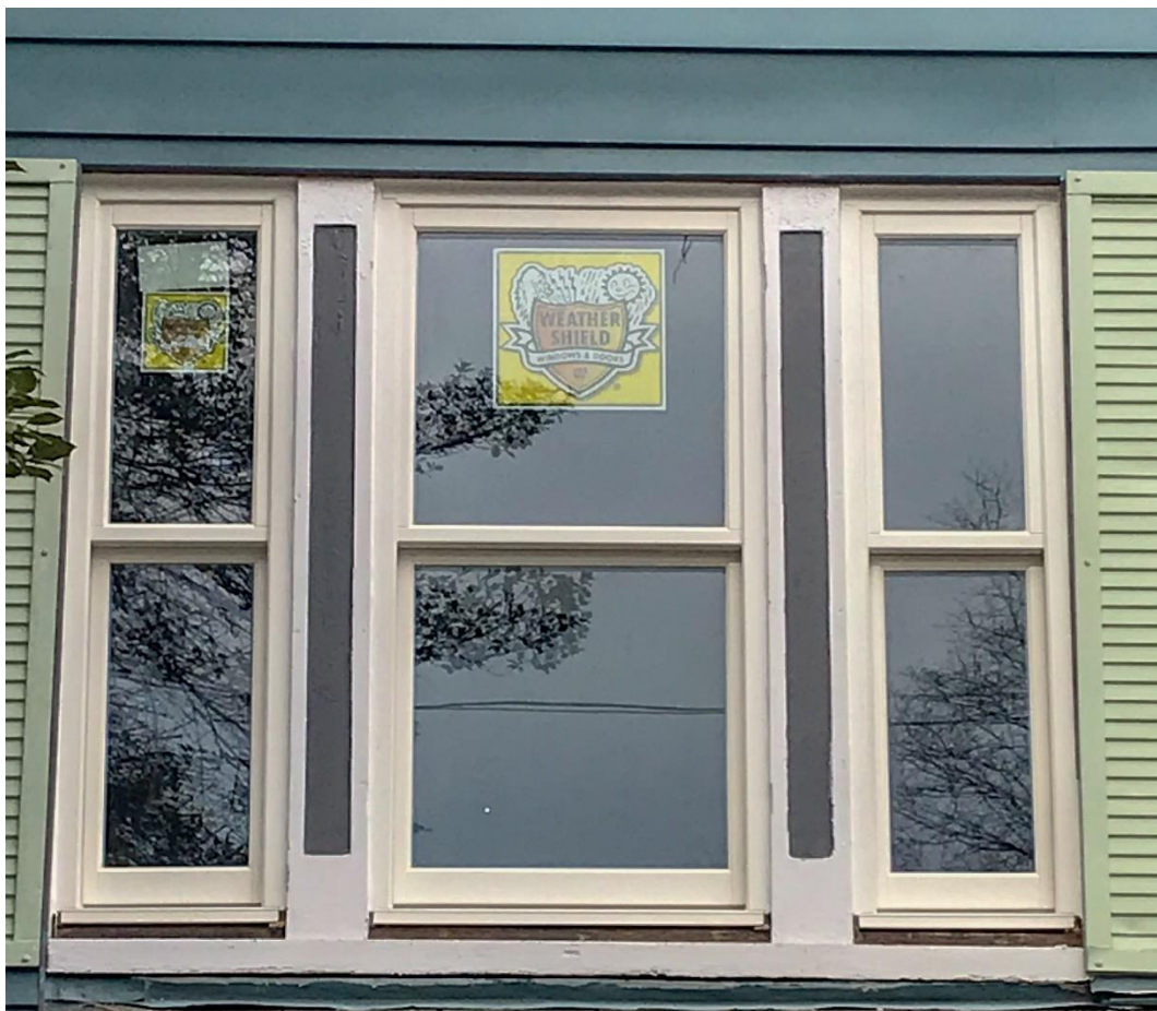
Figure 4: Detail showing the tri-partite sash window under the principal front-facing gable. The windows have been furred into the original framed openings with significant gaps where original trim was removed.
