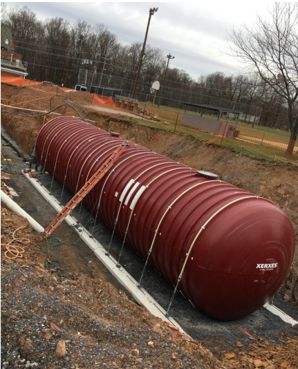
Figure 3.28: Underground water tanks may serve as additional fire protection measures where operational access is limited, such as on rural and rustic roads
