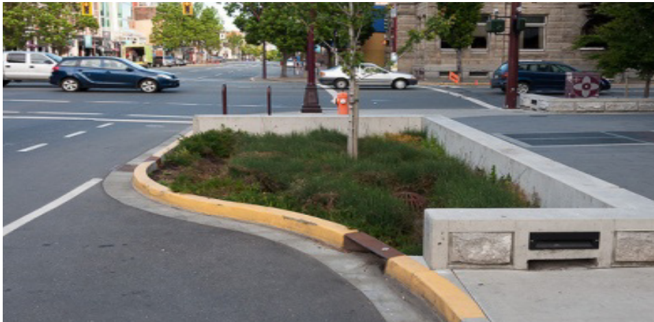
Figure 3.22: Curb extension create tighter corners and therefore reduces turning speeds of vehicles
