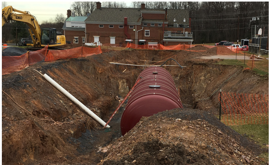
Figure 3.28: Underground water tanks may serve as additional fire protection measures where operational access is limited, such as on rural and rustic roads
