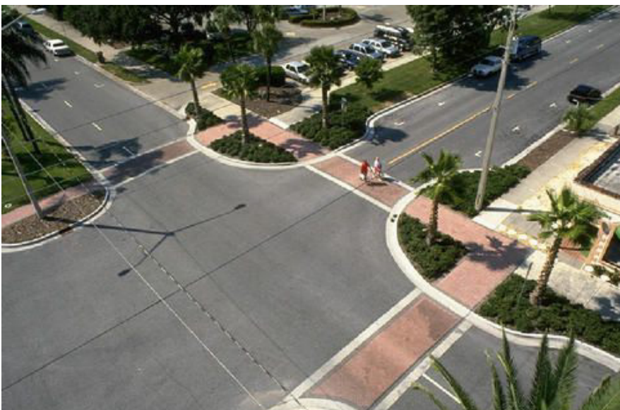
Figure 3.21: Bulb-outs create shorter crosswalk distance for pedestrians
