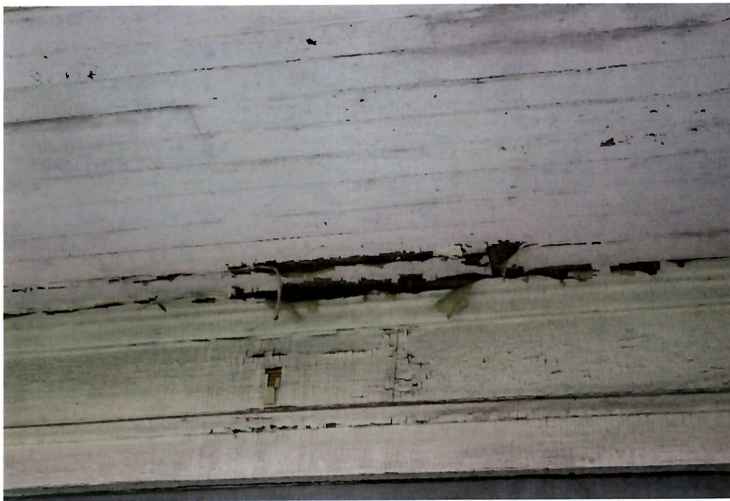
Photo 13. 08/05/19. Side (east). Project area. Detail of wood ceiling, trim, and molding to be repaired and painted.
