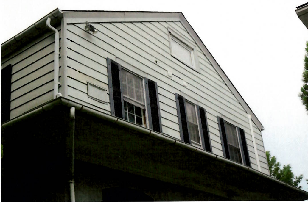
Photo 16. 08/05/19. Side (west) elevation. Project area. Center close-up showing aluminum siding to be removed; non-original shutters to be replaced and painted; wood ceiling, trim, and molding to be repaired and painted; stucco to be repaired and painted; aluminum gutters and downspouts to be repaired.
