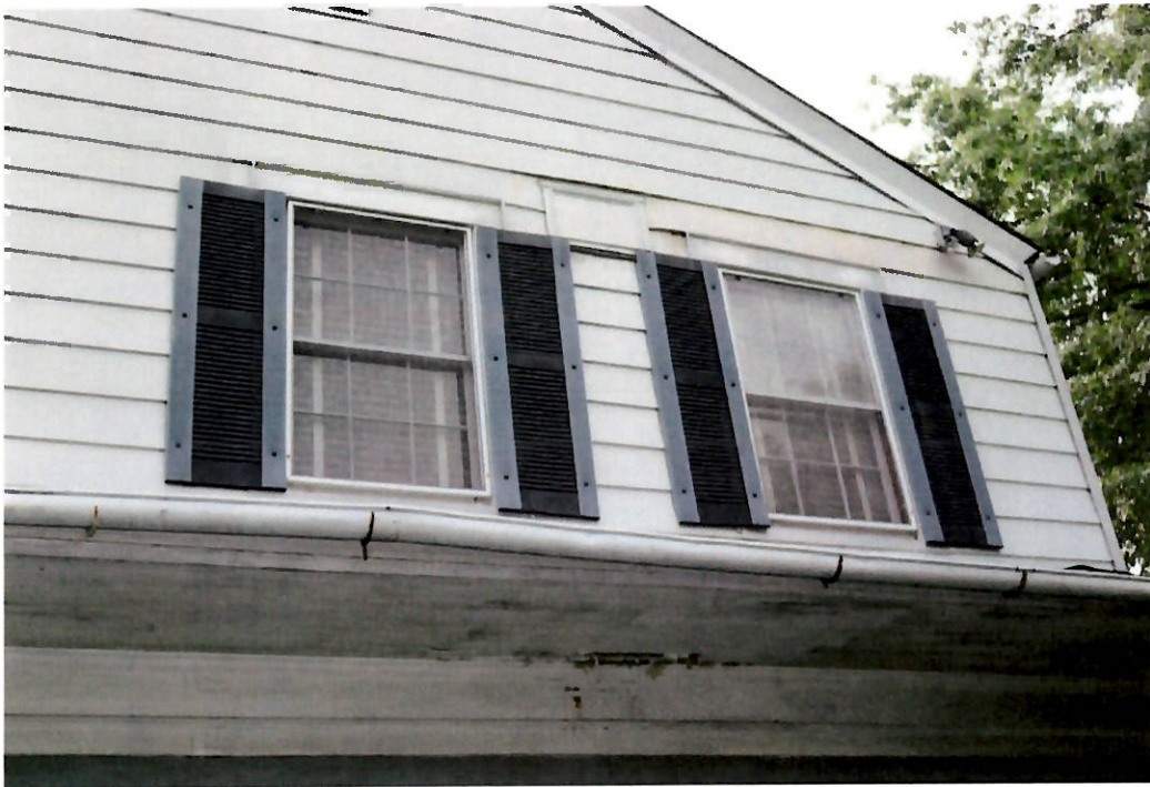
Photo 11. 08/05/19. Side (east) elevation. Project area. Right close-up showing aluminum siding to be removed; non-original shutters to be replaced and painted; wood ceiling, trim, and molding to be repaired and painted; aluminum gutters to be repaired.
