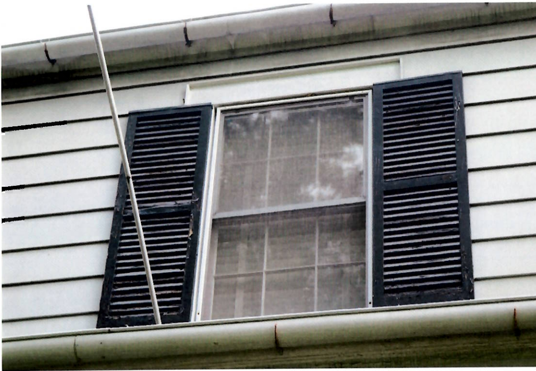
Photo 5. 08/05/19. Front (north) elevation. Project area. Detail of shutter to be restored and painted.
