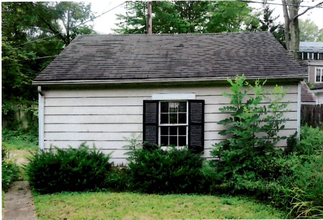
Photo 23. 08/05/19. Backyard (south). Garage. Project area. Close-up of north side of garage showing aluminum siding to be removed; shutters to be restored and painted; aluminum gutters and downspouts to be repaired.
