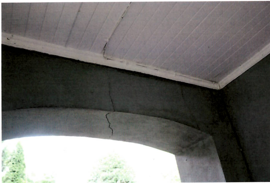
Photo 8. 08/05/19. Front (north). Project area. Porch. Detail of stucco to be repaired and painted.
