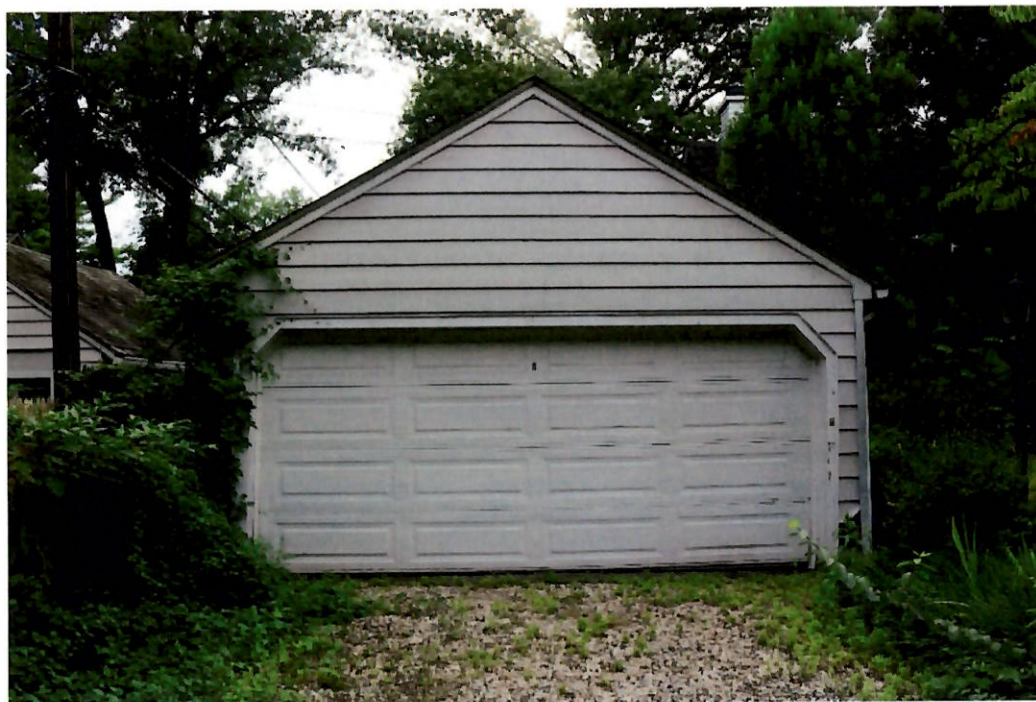
Photo 24. 08/05/19. Backyard (south). Garage. Project area. Close-up of east side of garage showing aluminum siding to be removed; aluminum gutters and downspouts to be repaired.
