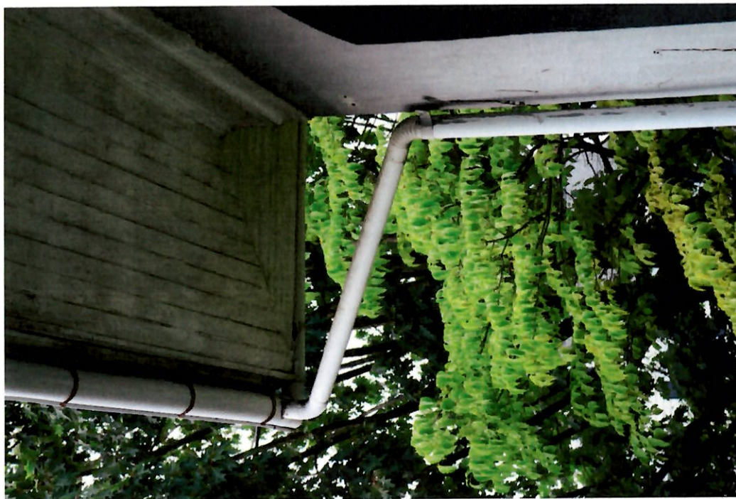
Photo 18. 08/05/19. Side (west). Project area. Detail of wood ceiling, trim, and molding to be repaired and painted; stucco to be repaired and painted; aluminum gutters and downspouts to be repaired.
