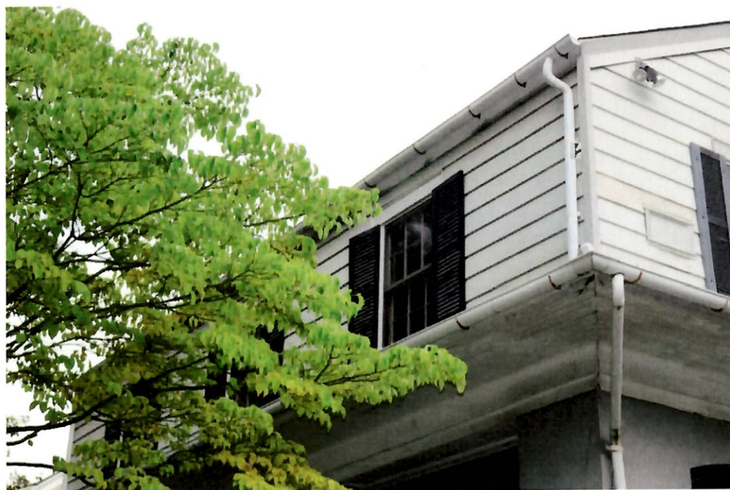
Photo 4. 08/05/19. Front (north) elevation. Project area. Right close-up showing aluminum siding to be removed; shutters to be restored and painted; wood porch ceiling, trim, and molding to be repaired and painted; stucco to be repaired and painted; aluminum gutters and downspouts to be repaired.
