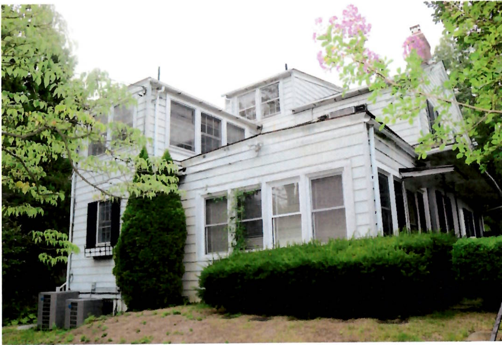
Photo 21. 08/05/19. Back (south) elevation. Project area. Right close-up showing aluminum siding to be painted; shutters to be painted; aluminum gutters and downspouts to be repaired.
