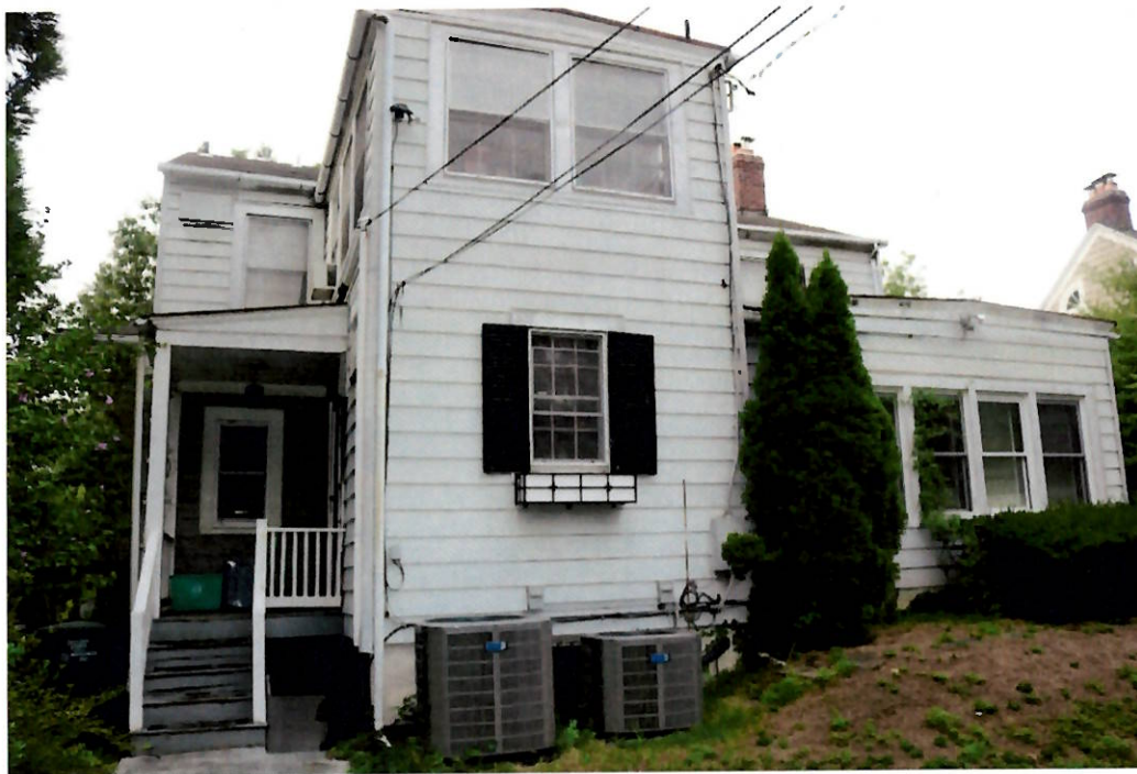
Photo 20. 08/05/19. Back (south) elevation. Project area. Left close-up showing aluminum siding to be painted; shutters to be painted; wood ceiling, trim, and molding to be painted; aluminum gutters and downspouts to be repaired.
