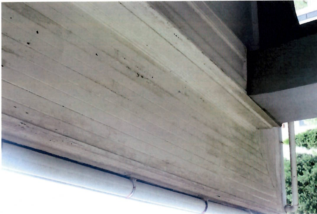
Photo 7. 08/05/19. Front (north). Project area. Porch. Detail of wood porch ceiling, trim, and molding to be repaired and painted; aluminum gutters and downspouts to be repaired.
