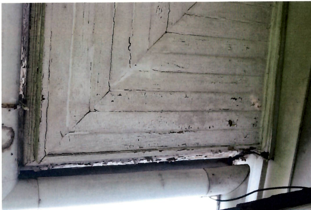
Photo 14. 08/05/19. Side (east). Project area. Detail of wood ceiling, trim, and molding to be repaired and painted; aluminum gutters to be repaired.
