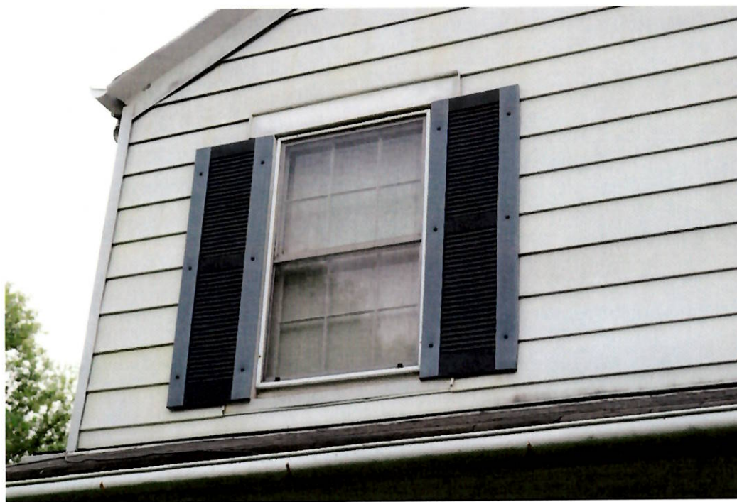
Photo 10. 08/05/19. Side (east) elevation. Project area. Left close-up showing aluminum siding to be removed; non-original shutters to be replaced and painted; aluminum gutters to be repaired.
