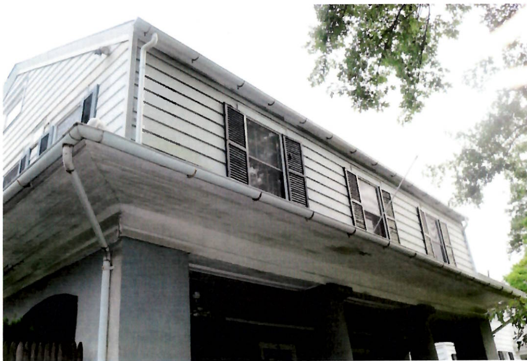
Photo 3. 08/05/19. Front (north) elevation. Project area. Left close-up showing aluminum siding to be removed; shutters to be restored and painted; wood porch ceiling, trim, and molding to be repaired and painted; stucco to be repaired and painted; aluminum gutters and downspouts to be repaired.
