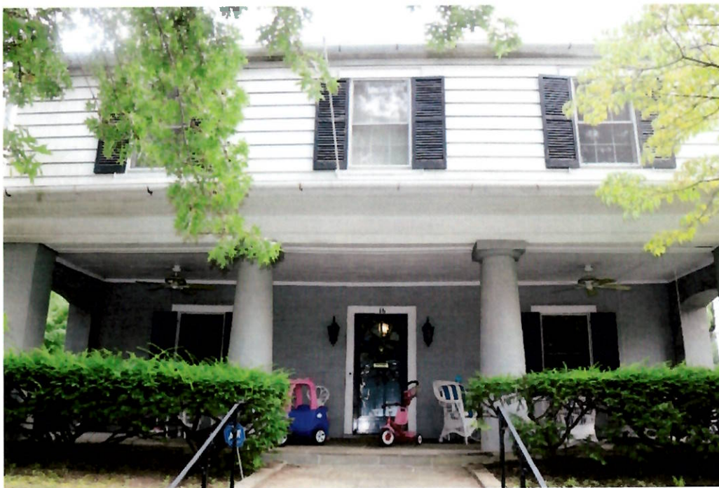
Photo 2. 08/05/19. Front (north) elevation. Project area. Center close-up showing aluminum siding to be removed; shutters to be restored and painted; wood porch ceiling, trim, and molding to be repaired and painted; stucco to be repaired and painted; aluminum gutters to be repaired.
