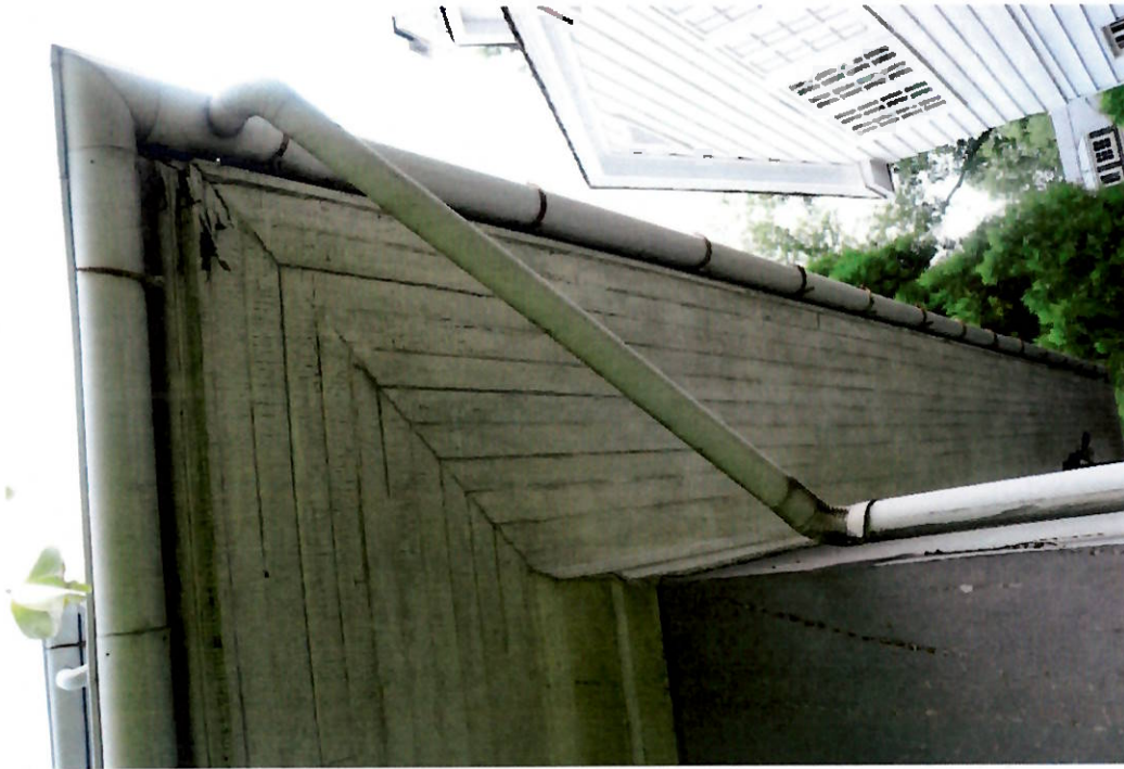
Photo 17. 08/05/19. Side (west). Project area. Detail of wood ceiling, trim, and molding to be repaired and painted; stucco to be repaired and painted; aluminum gutters and downspouts to be repaired.
