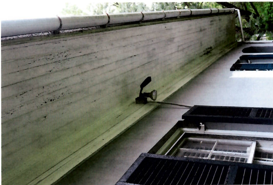
Photo 12. 08/05/19. Side (east). Project area. Detail of shutters to be restored and painted; wood ceiling, trim, and molding to be repaired and painted; stucco to be repaired and painted; aluminum gutters and downspouts to be repaired.
