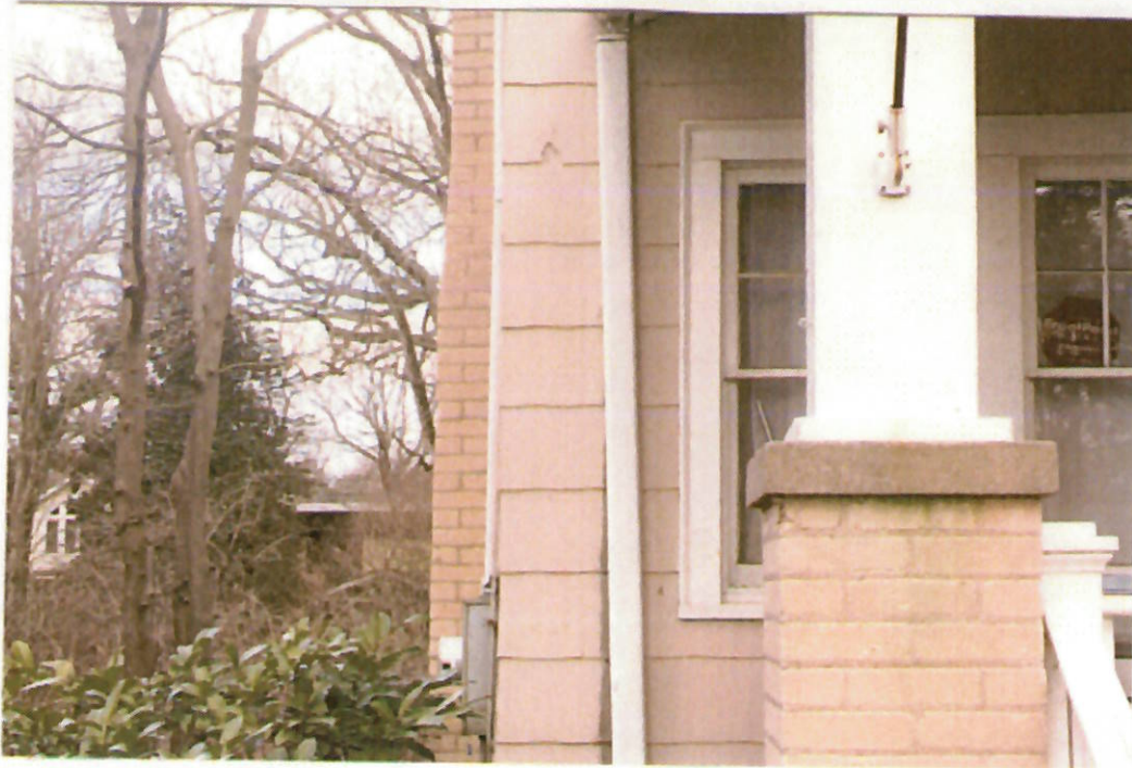
Detail: BROKEN DOWNSPOUTS
