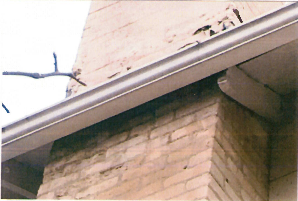
Detail: CHIMNEY DETERIORATING, BROKEN EAVE
