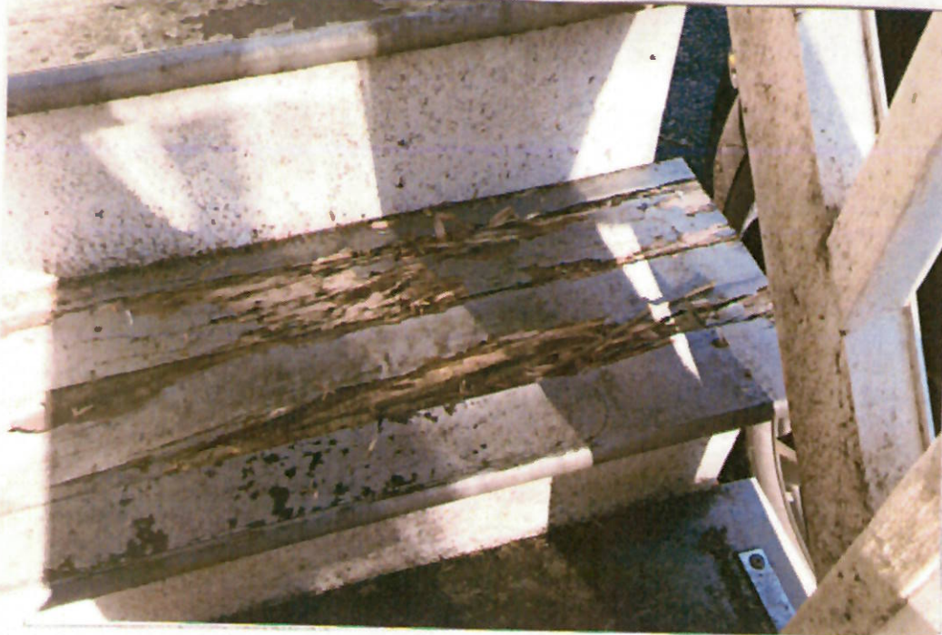
Detail: SIDE PORCH BROKEN/ROTTING STEPS
