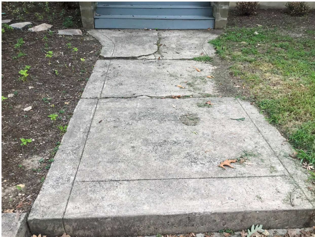
Figure 3: The existing, cracked front walk.
