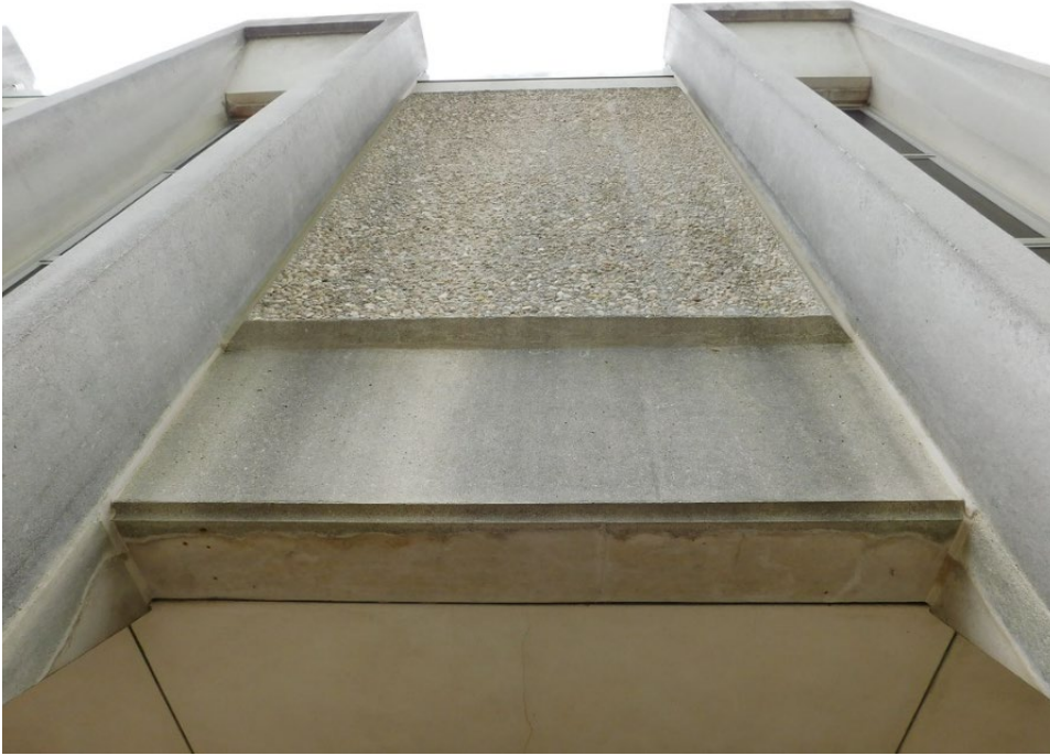
Figure 9: Detailed view of second-story windows and exposed aggregate panel.
