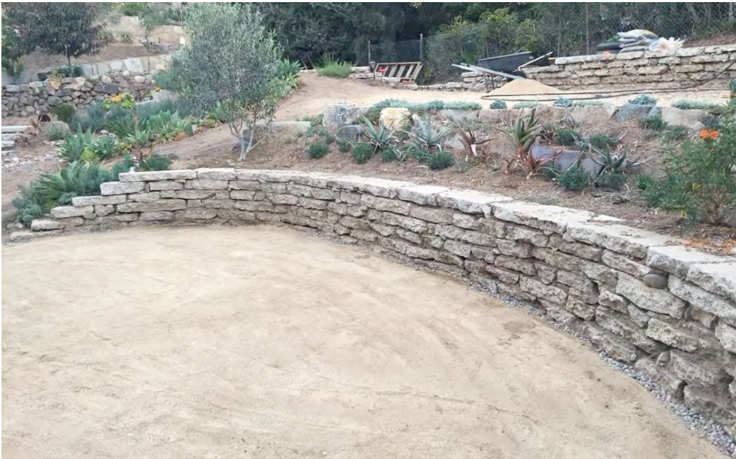
Figure 6—Example of recycled concrete wall. Proposed as option for lower replacement wall.
