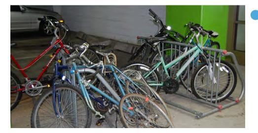
Schoolyard racks (top) and wave racks (bottom) do not support a bicycle with two points of contact leading to inefficient, haphazard parking that can damage bicycles.
