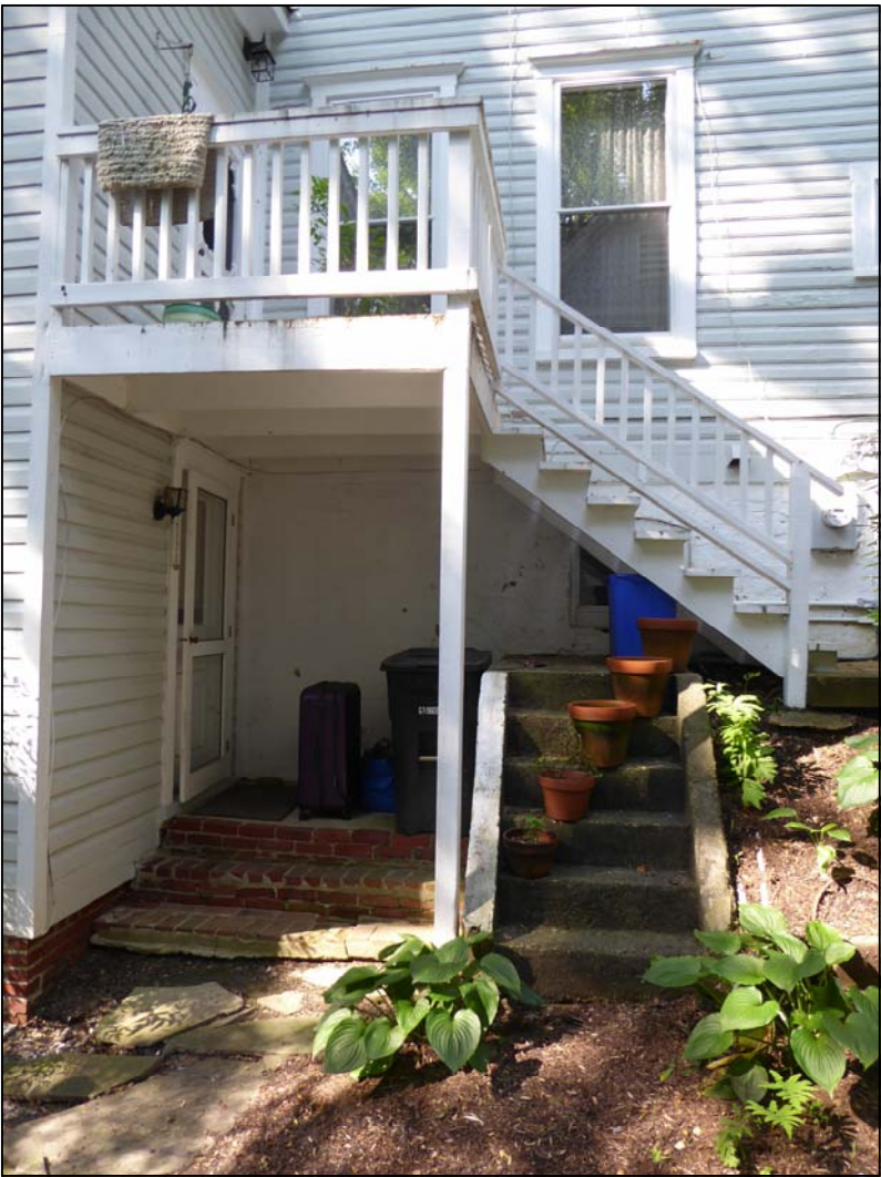
NORTH -EAST SIDE: REMOVE AND INFILL EXISTING WINDOW BEHIND STEPS (NOT ORIGINAL TO THE HISTORIC HOUSE)
