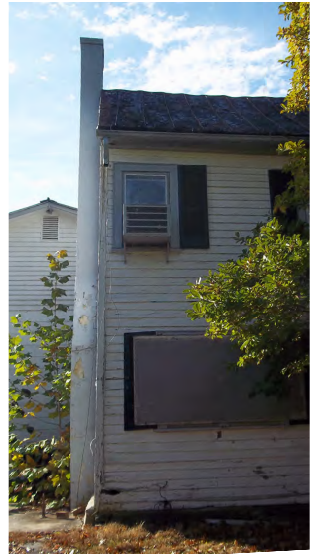
NORTH ELEVATION OF EAST CHIMNEY SHOWING 16 INCH WIDTH
