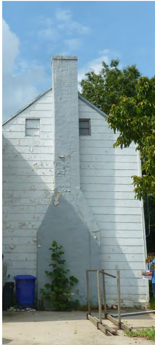
EAST ELEVATION OF EAST CHIMNEY SHOWING ADDED BRICK VENT TO NORTH
