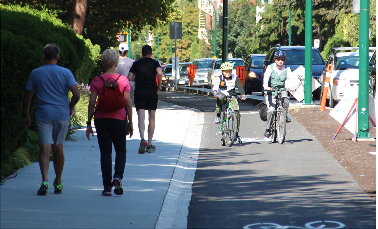
A landscaped buffer will provide separation from traffic on this separated bike lane at an intermediate level between the street and sidewalk in Vancouver, British Columbia, Canada.
