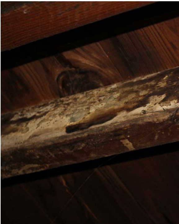
FIGURE 82 Termite damage evident in attic.
