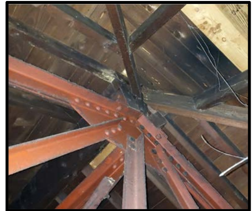
Figure 10 – Hip Connection
