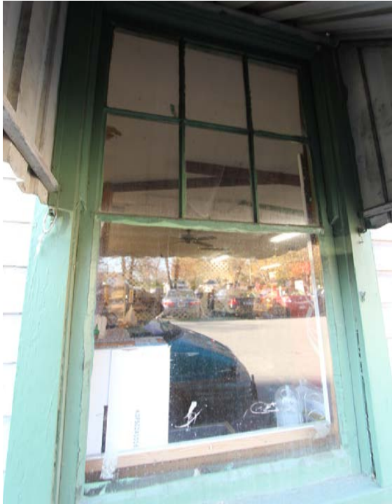
FIGURE 44 Extant window missing lower muntins.
