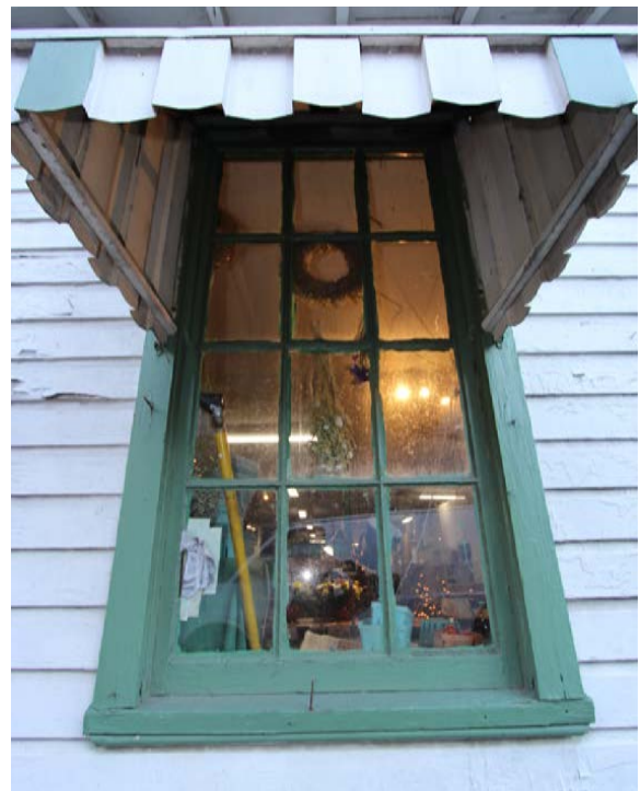
FIGURE 21 Original twelve-light, wood-sash pivot window.
