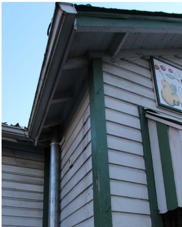
FIGURE 20 Detail of wood trim, overhanging eave with exposed rafter tails, and addition of gutter and downspout.
