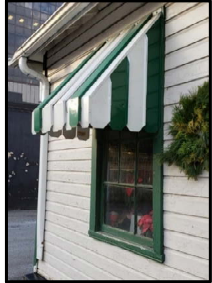
Figure 12 – Cold formed Steel Awnings
