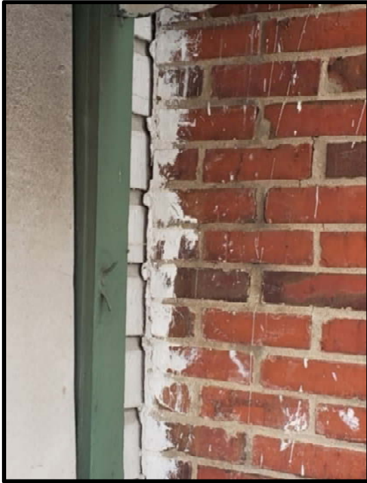
Figure 16 – Visible Gap Between Buildings and Chimney
