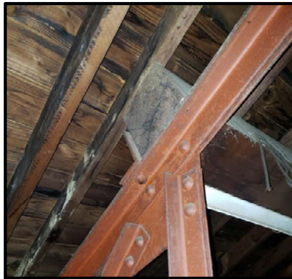
Figure 8 – Typical Beam Support
