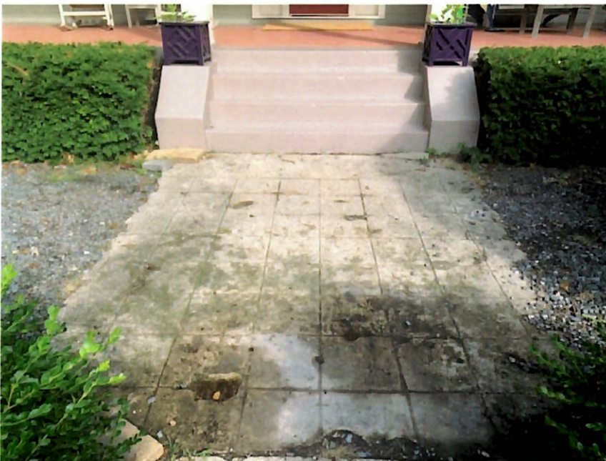
(2) EXISTING CONCRETE AREA SHOWN HERE TO BE REPLACED BECAUSE IT IS IN POOR CONDITION. REPLACEMENT MATERIALS ARE THE HISTORIC "TERRA COTTA" PAVERS THAT WERE USED ON OUR SIDEWALKS
