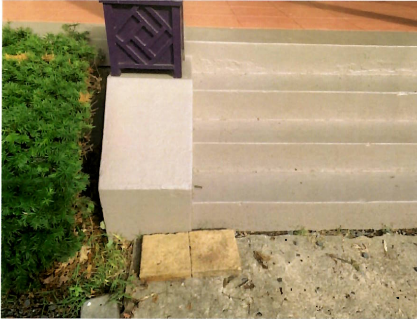
(3) HISTORIC PAVERS SHOWN HERE ARE TO REPLACE THE CONCRETE
