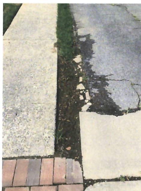
View of erosion between driveways
