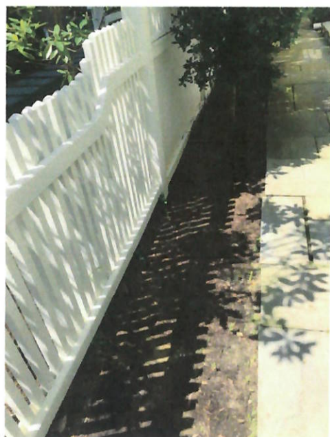
View of erosion behind front fence
